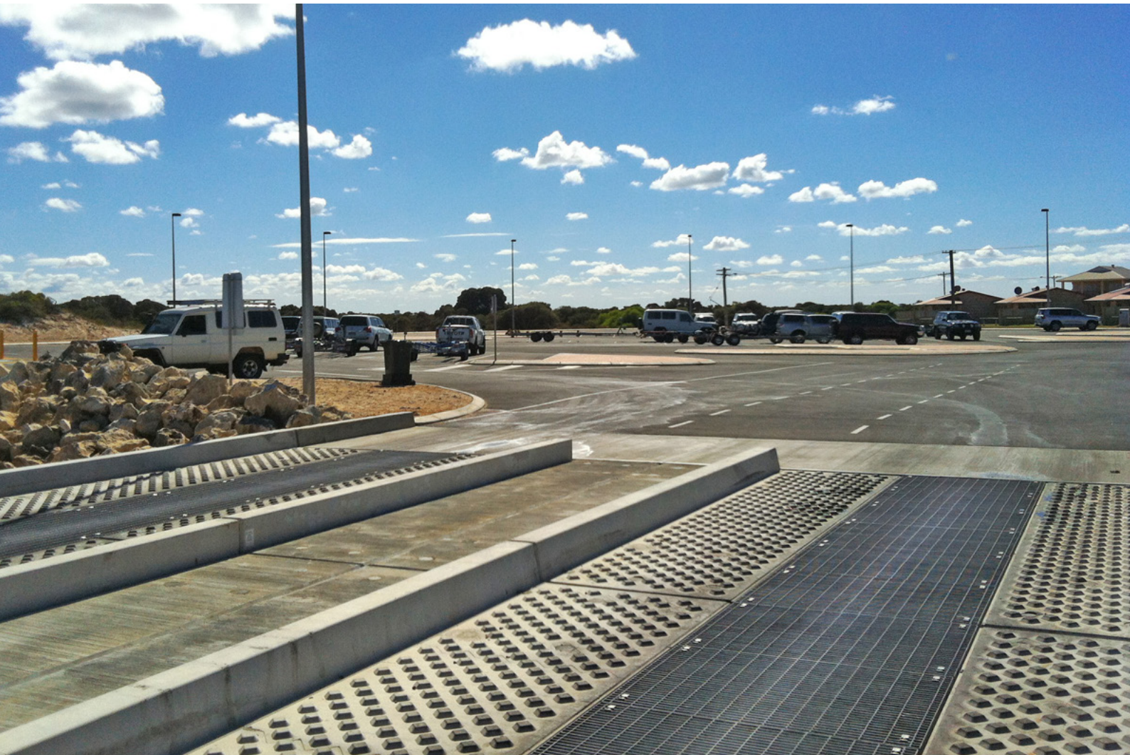
Illyarrie Street boat ramp, Shire of Coorow
