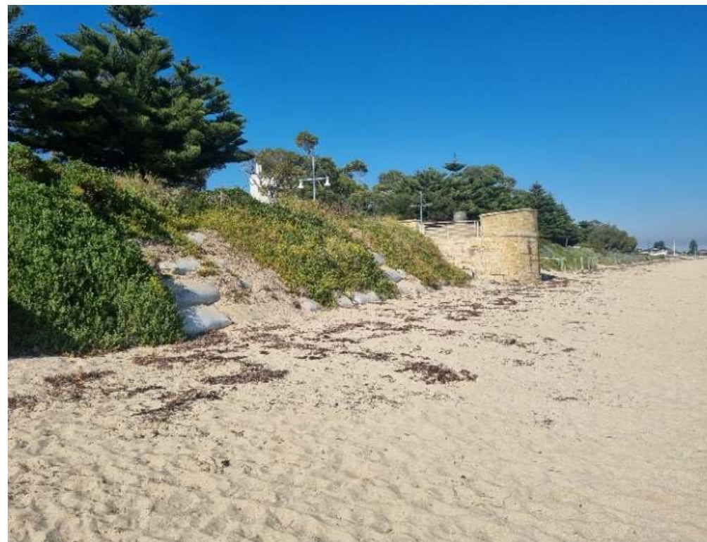
Figure 8-4: Photo taken of revegetation above Flinders Ln GSC seawall, approximate chainage +3350 m. Taken during site visit 18 September 2024.
