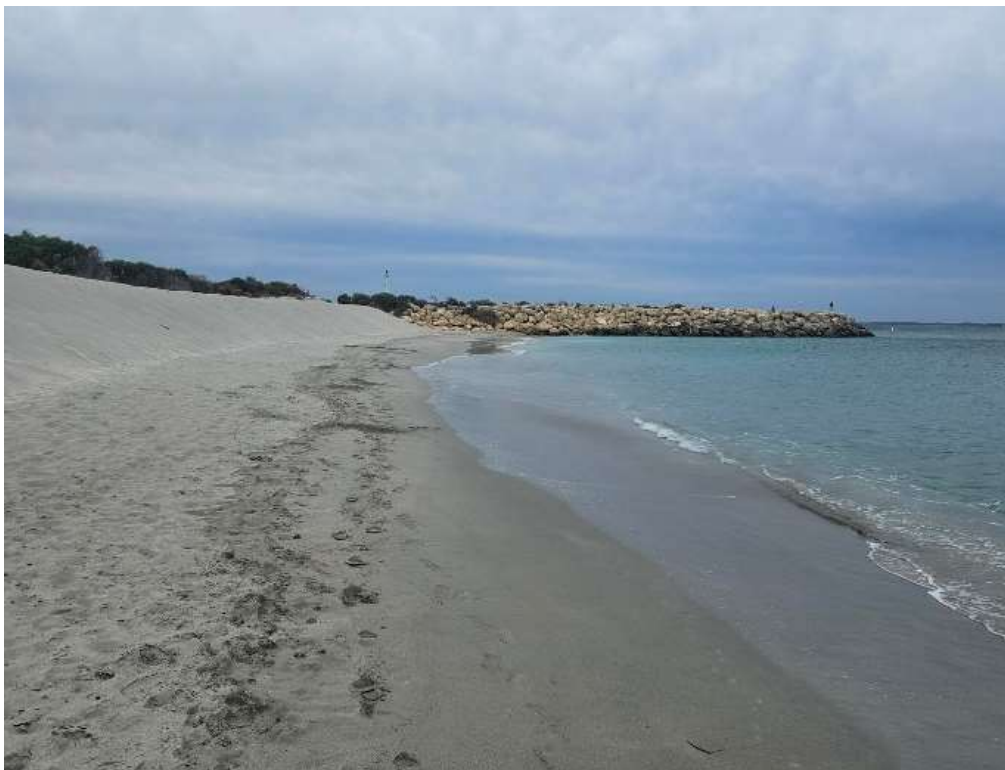
Figure 5-7: Catherine Point Groyne and beach dune/beach profile, looking south (taken during site visit 9 May 2024)
