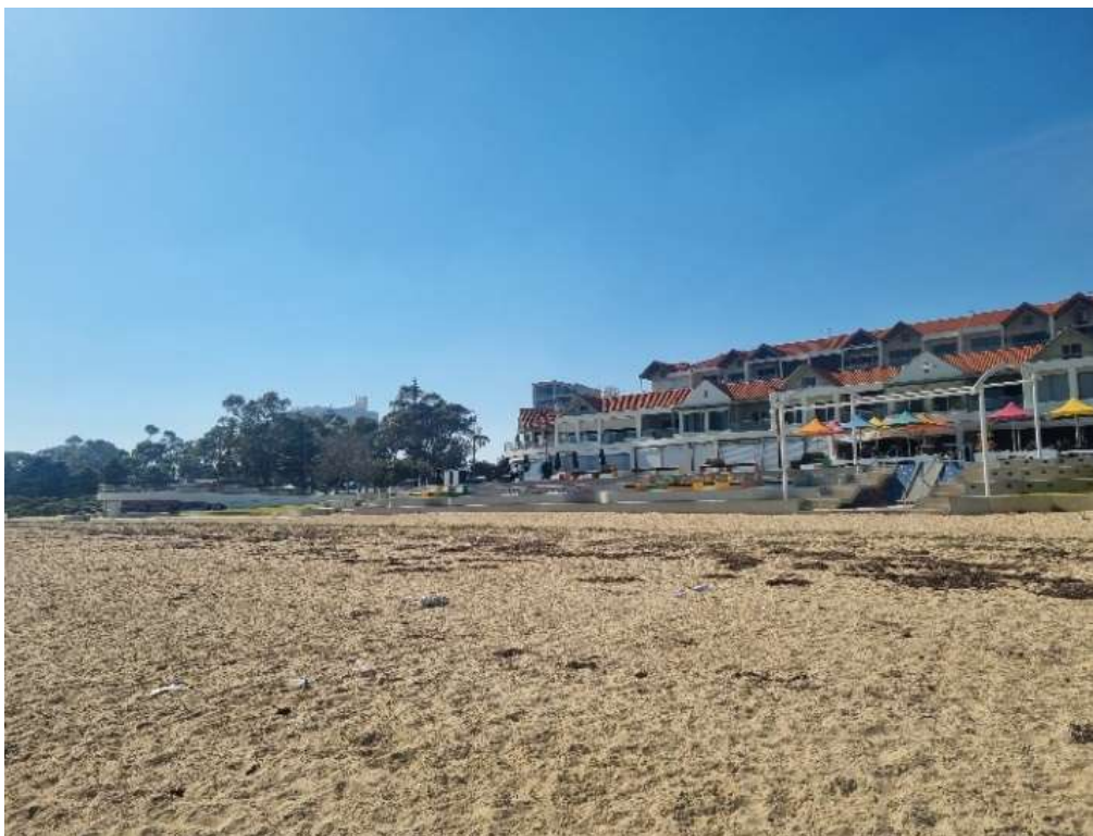
Figure 8-9: Val St. foreshore concrete retaining structures (+2925m). Taken during site visit 18 September 2024.
