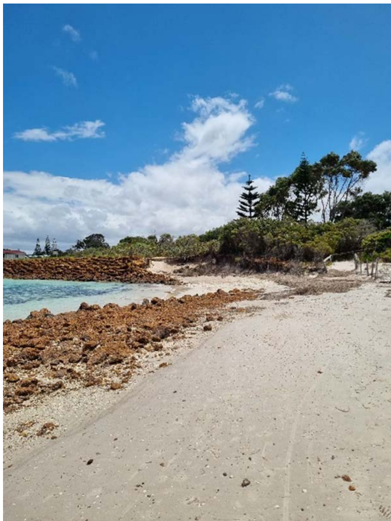
Figure 12-11: Exposed rock along artificial headland tombolo. Damaged seawall and dune erosion in background. Taken facing northwest during site visit 5 December 2024
