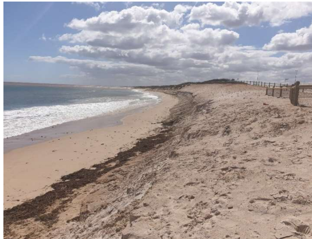
Figure 1-3: Photo taken of Surf Beach dune/beach profile, post storm event, scarp and exposed concrete face apparent 11 April 2021
