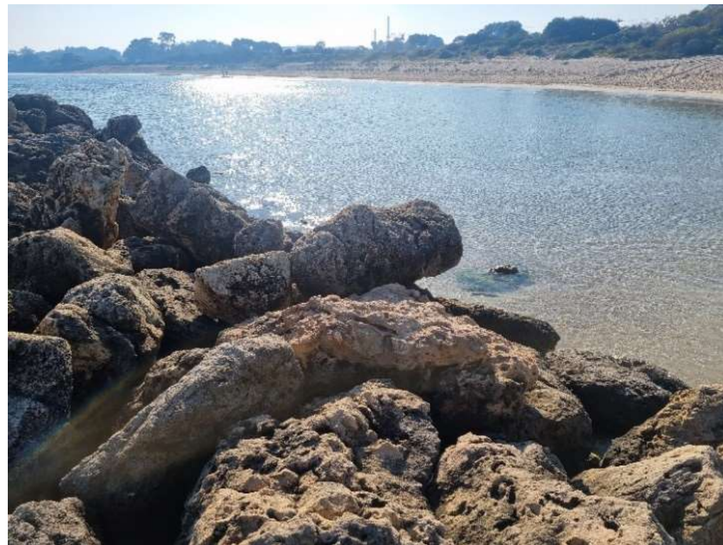
Figure 7-16: Southern artificial headland, taken from crest, during site visit 18/09/2024.
