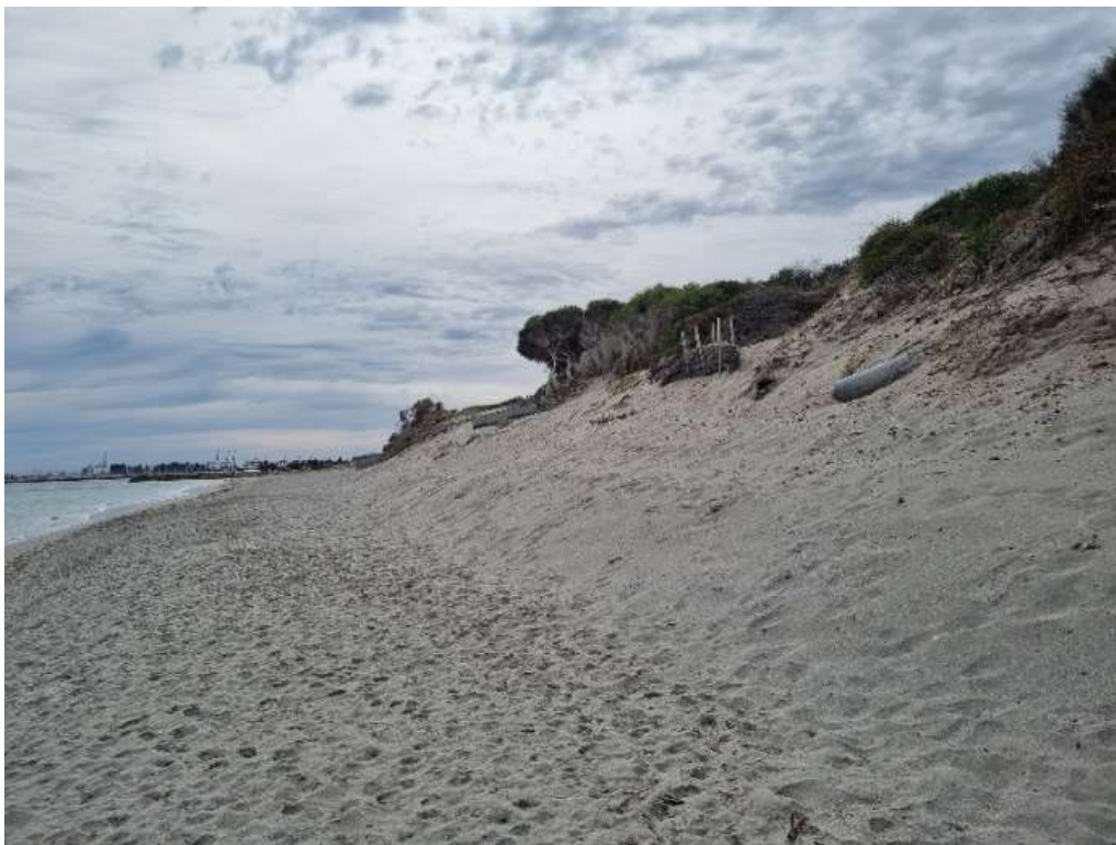
Figure 5-3: Photo taken of C.Y. O'Connor beach dune/beach profile (north of Catherine Point Groyne), during site visit 9 May 2024
