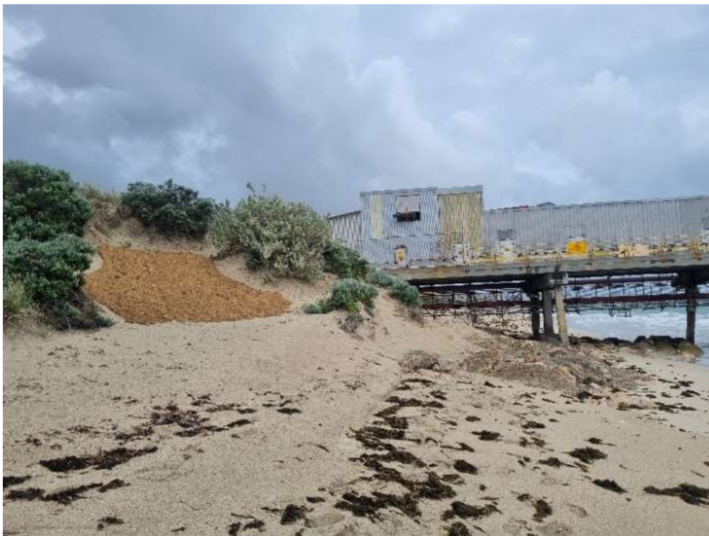
Figure 6-13: Jute matting stabilisation installed directly north of Alcoa Jetty, taken during site visit 14 August 2024.
