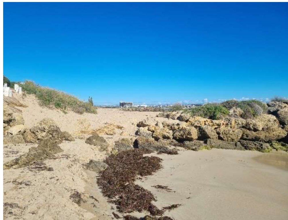
Figure 10-4: Scattered armour transition between Groyne 2 (Henson St.) neck and dune system. Taken facing south-west during site visit 1 July 2024.
