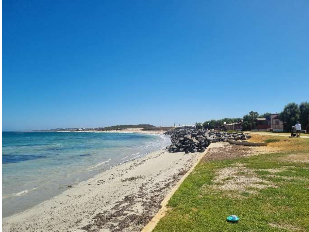
Figure 1-8: Seawall and retaining wall looking north (taken during site visit 29 January 2024)
