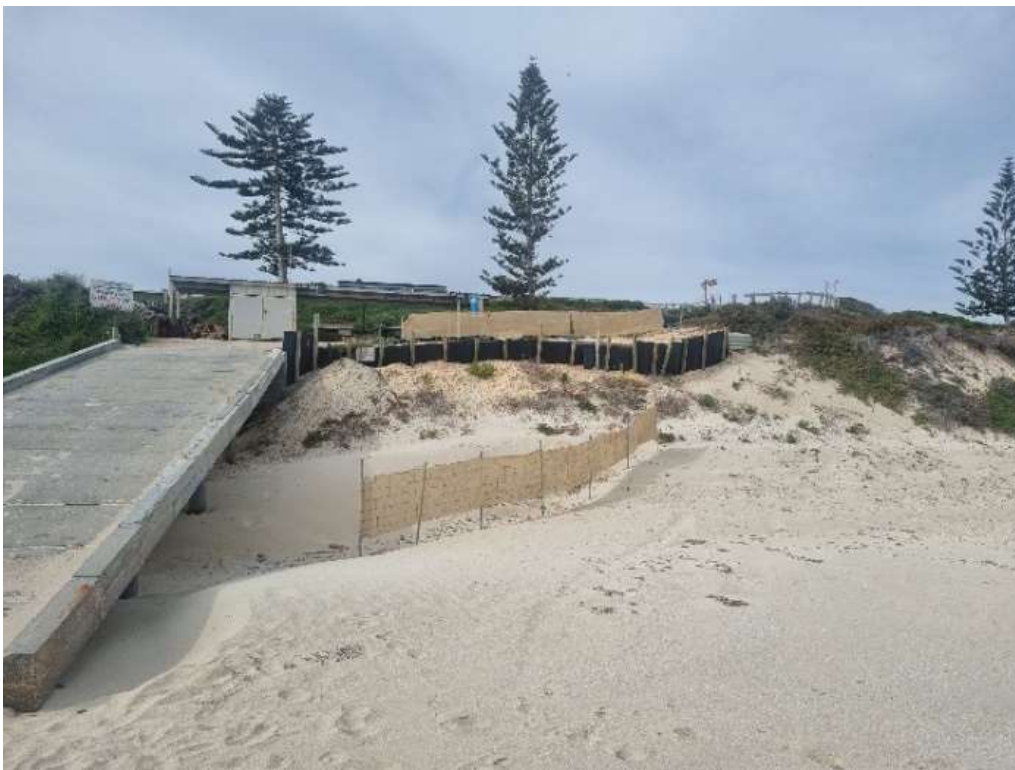
Figure 3-6: Seabird Private Caravan Park, private access vehicle ramp. Light retaining structure and wind fencing in place to protect road access. Facing east, taken during site visit 20 May 2024.
