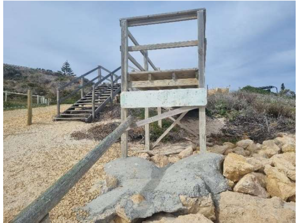
Figure 3-5: Pedestrian boardwalk/lookout at the Edwards St beach access ramp. northern terminus of the rock revetment. Concrete foundations exposed indicating likely erosion since initial construction. Photo taken facing south-east during site visit 20 May 2024.
