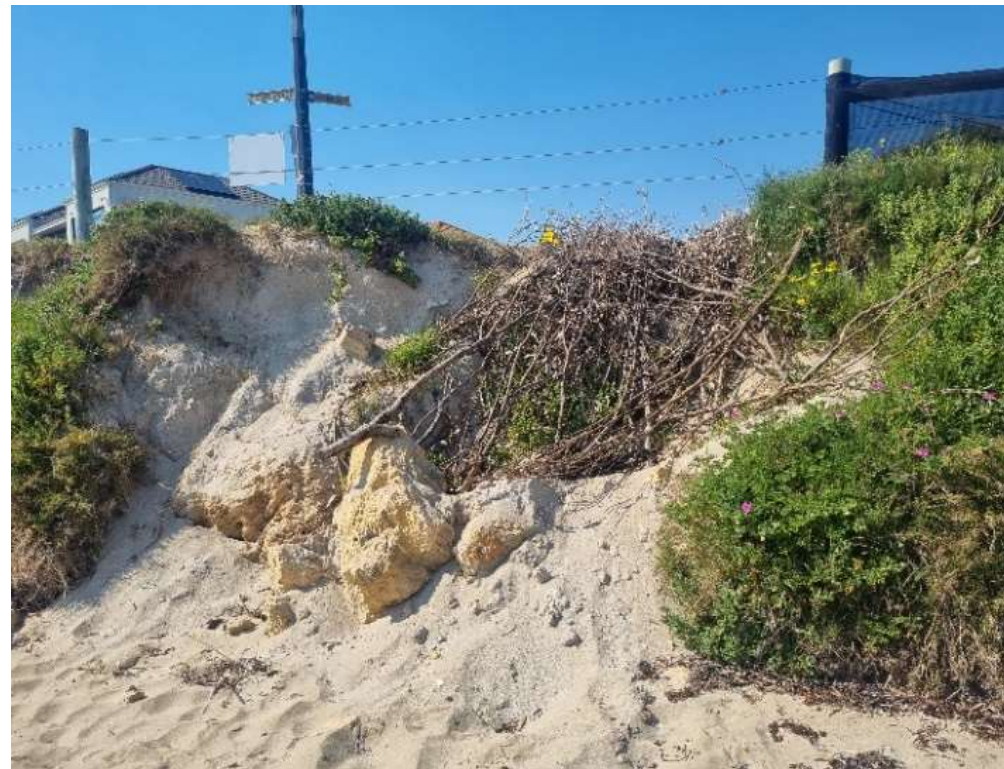
Figure 8-18: Brushing applied to erosion at Hymus St. informal seawall (+1375m). Taken during site visit 18 September 2024.
