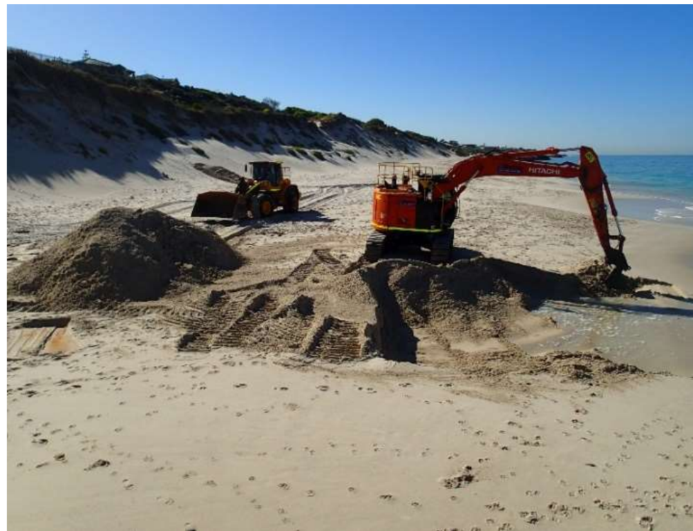
Figure 4-6: 'Scraping' sand from swash zone adjacent to Groyne 4, north end of Section 5, facing south (Ellyard, 2023)
