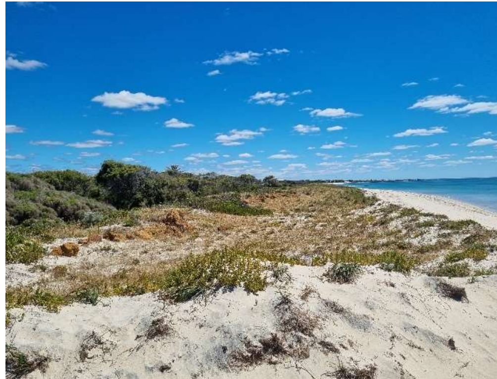
Figure 11-18: Buried informal seawall behind primary dune (+1800m), taken during site visit 27 November 2024.
