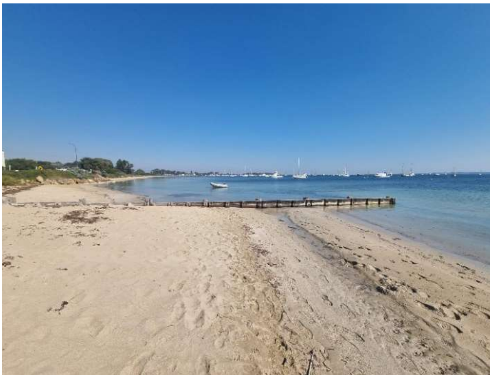
Figure 8-13: Hymus St. timber groyne and informal seawall (+1375m). Taken during site visit 18 September 2024.
