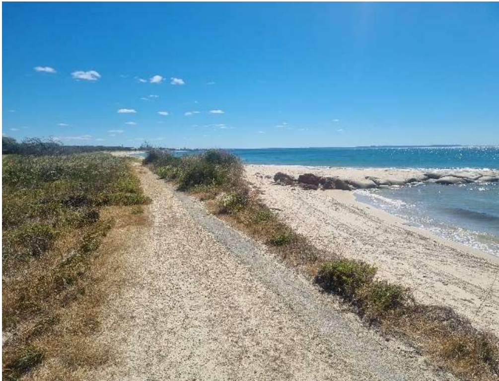
Figure 11-23: Eroded access track immediately north of groyne 10 (+1260m) taken during site visit 27 November 2024.
