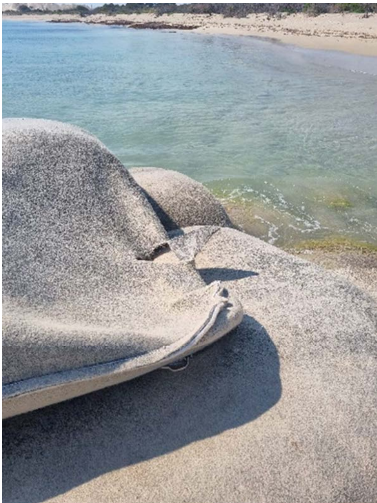
Figure 9-3: Ripped bags at neck end of GSC groyne. Taken during site visit 18 September 2024.
