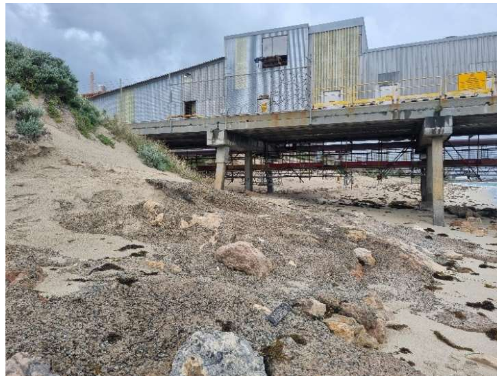
Figure 6-14: Cement stabilisation of beach directly north of Alcoa Jetty, taken during site visit 14 August 2024.
