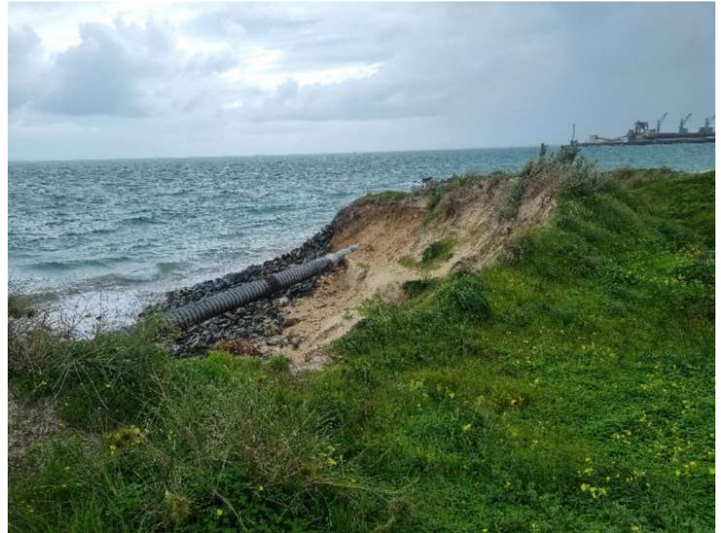
Figure 6-8: BP refinery storm water outfall, and scarping above (chainage +3250) taken facing northwest during site visit 14 August 2024.
