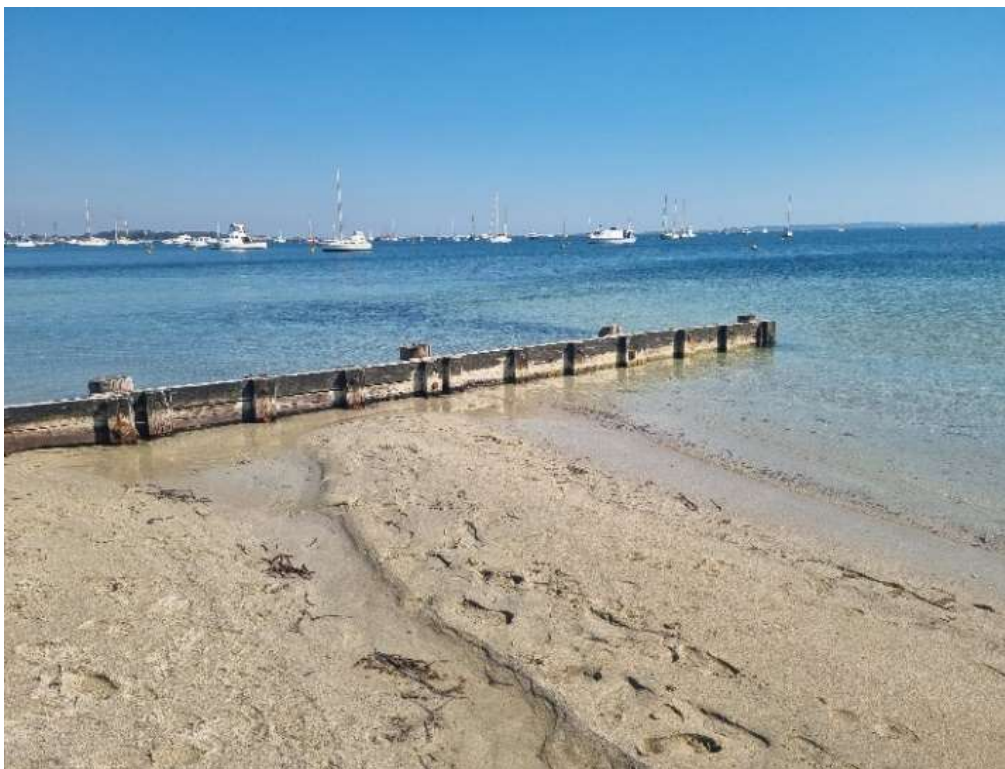
Figure 8-11: Hymus St. timber groyne (+1350m). Taken during site visit 18 September 2024.
