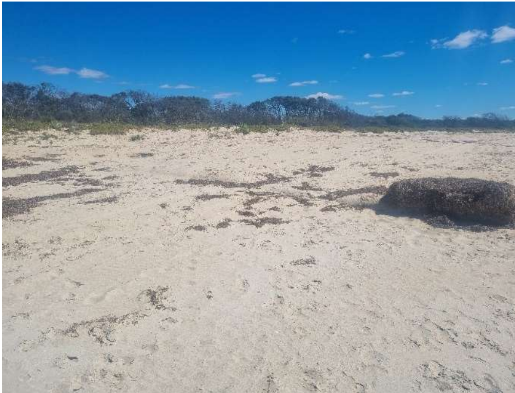
Figure 11-19: GSC Groyne 8, exposed bags driven over by four-wheel-drives taken during site visit 27 November 2024.
