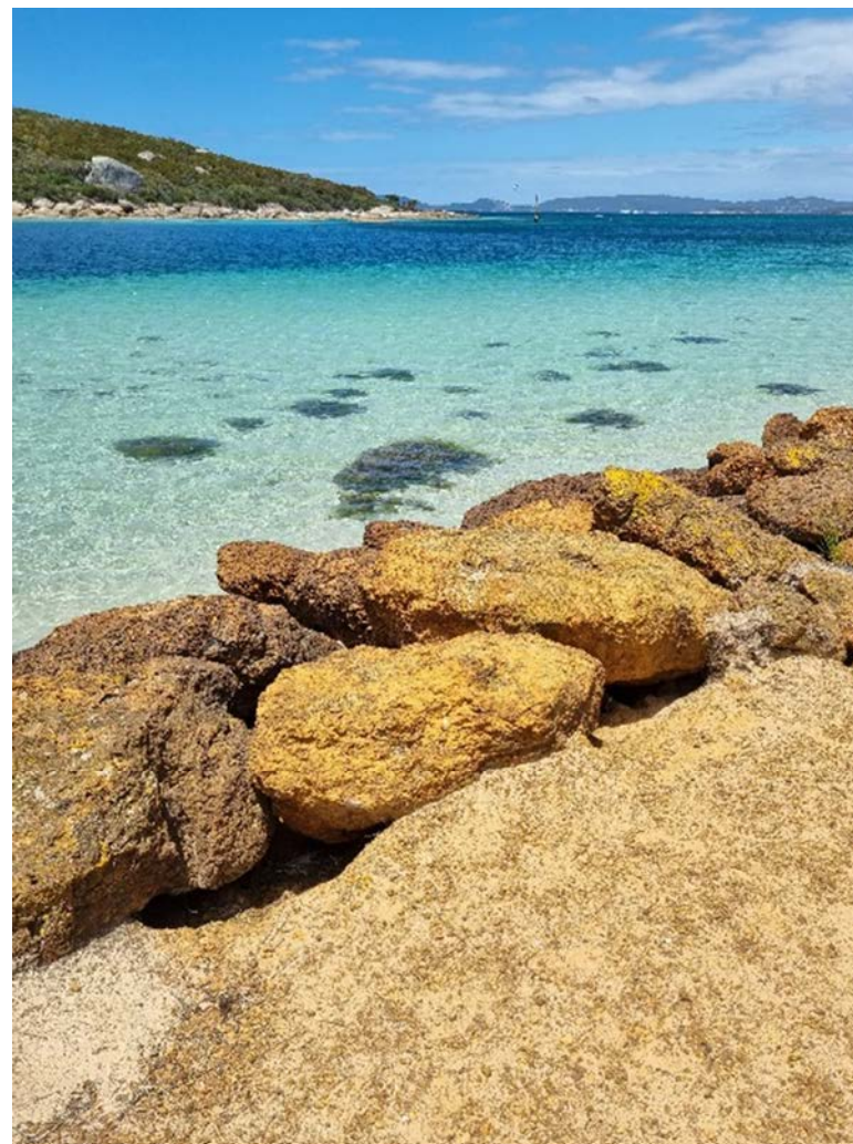
Figure 12-6: Scattered armour offshore of training wall. Taken facing south during site visit 5 December 2024.
