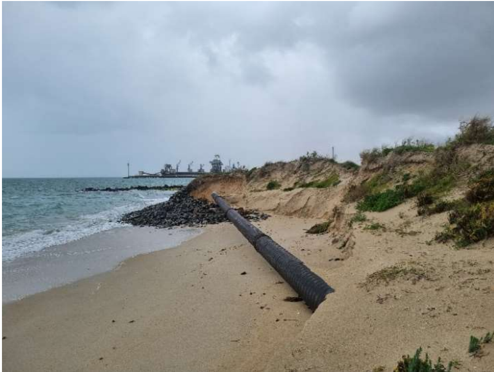
Figure 6-7: BP refinery storm water outfall, and informal armouring (chainage +3200) taken facing north during site visit 14 August 2024.
