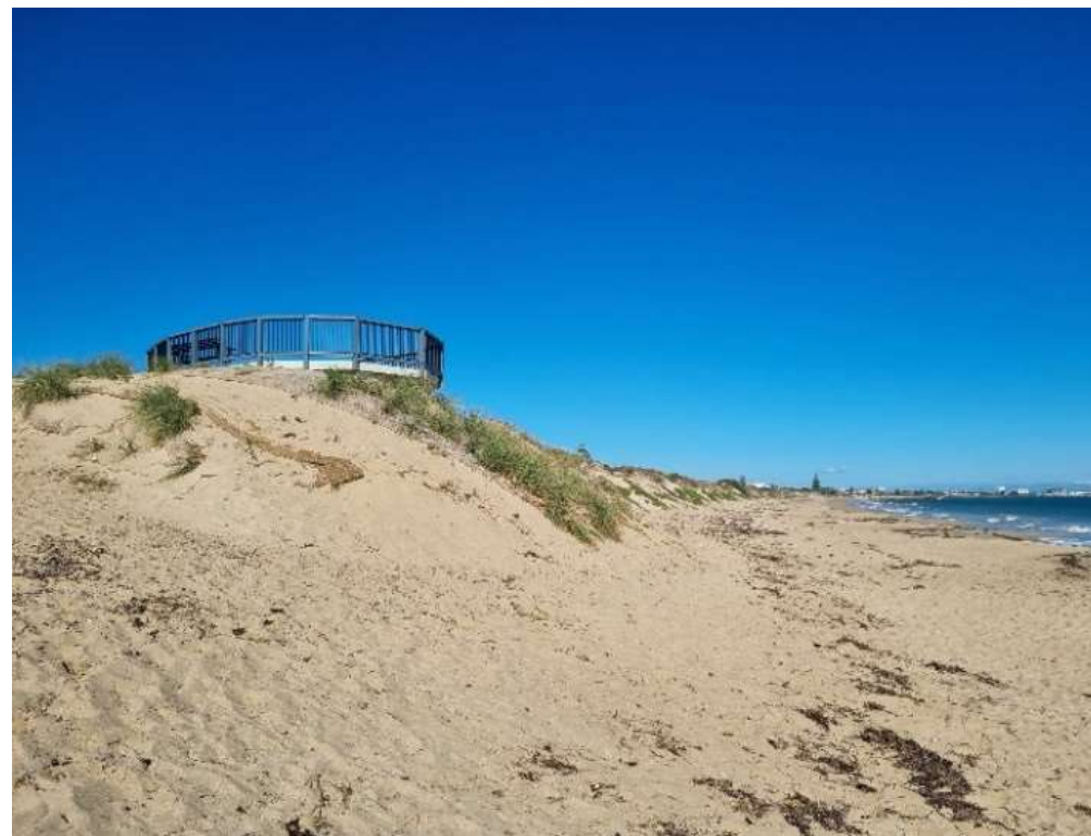
Figure 10-8: Watersun beach lookout, dune stabilisation works recently completed. Taken facing south during site visit 1 July 2024.
