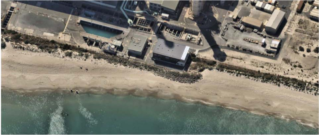
Figure 6-19: Oblique imagery of seawall adjacent to Synergy office and Kwinana Power Station. Nearmap imagery captured 15 October 2023.
