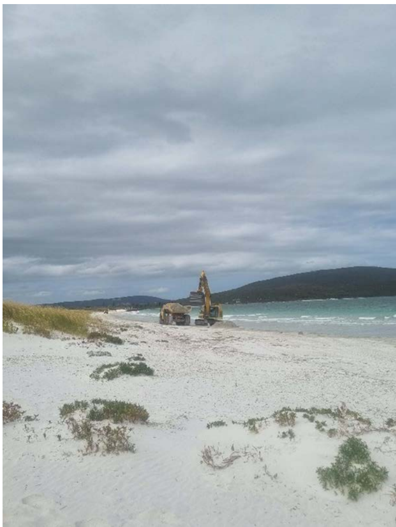
Figure 12-19: Sand nourishment works (excavation) at Griffiths St beach access (+2000m), taken during site visit 5 December 2024.
