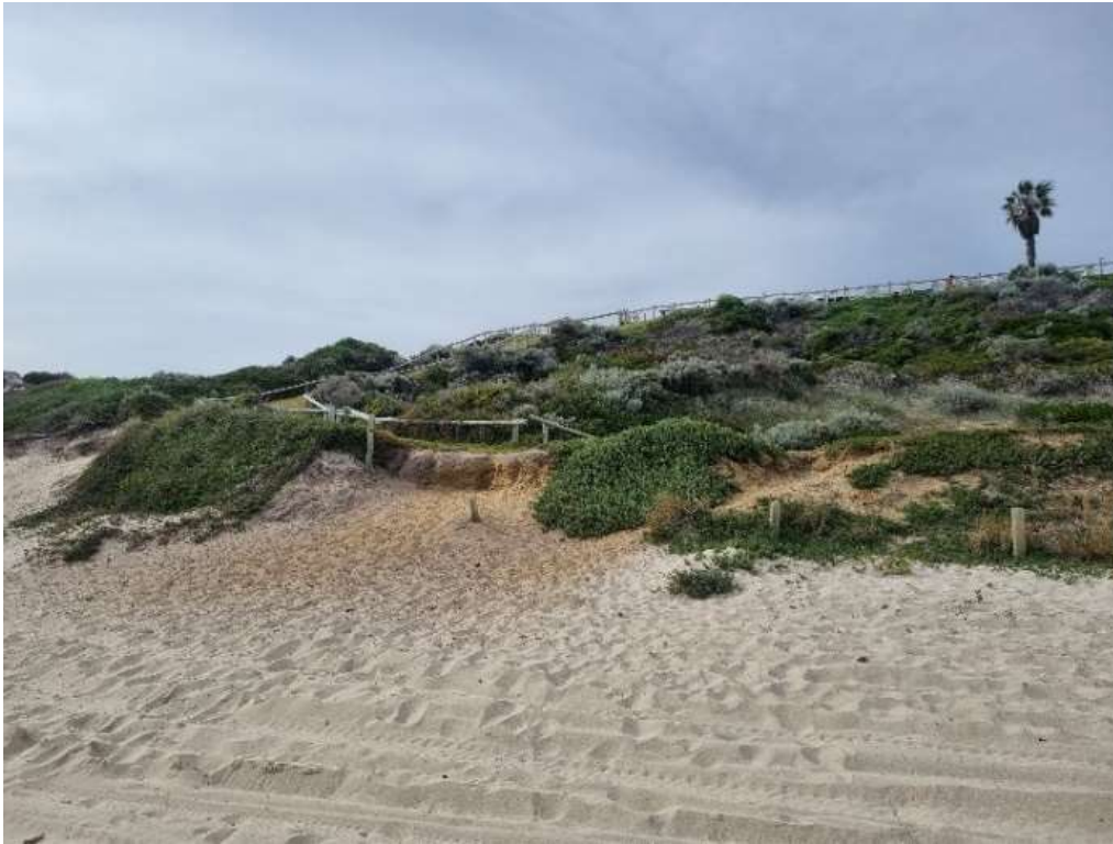
Figure 3-4: Private pedestrian access down from Seabird Tavern onto beach. Erosion apparent at base of access path. Taken facing east during site visit 20 May 2024.
