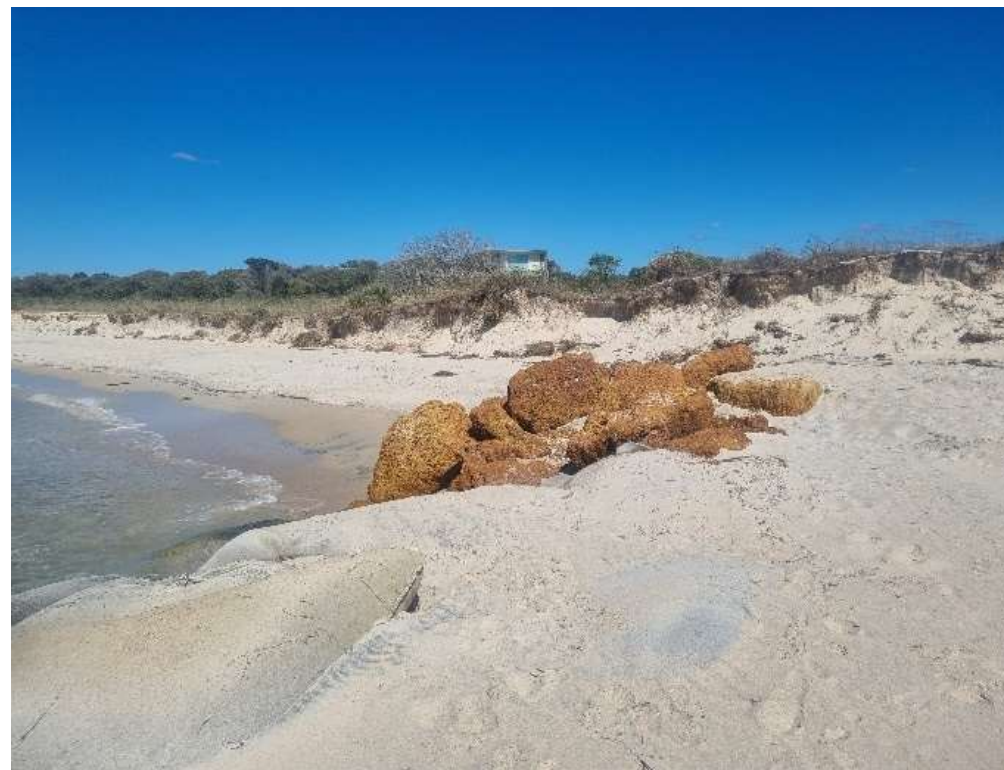
Figure 11-22: Informal groyne extension with laterite armouring at Groyne 10 (+1240m) taken during site visit 27 November 2024.
