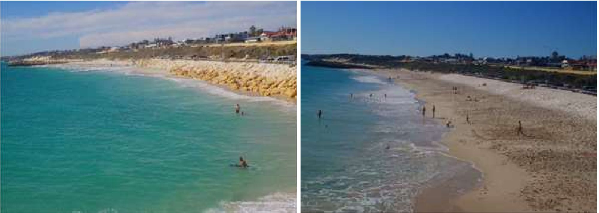
Figure 4-2: Photos taken from Groyne 1 fixed monitoring camera, looking north towards Section 3 (left) 30 January 2023 (right) 26 August 2023. Images show the extremes of seasonal morphological changes adjacent to the carpark.
