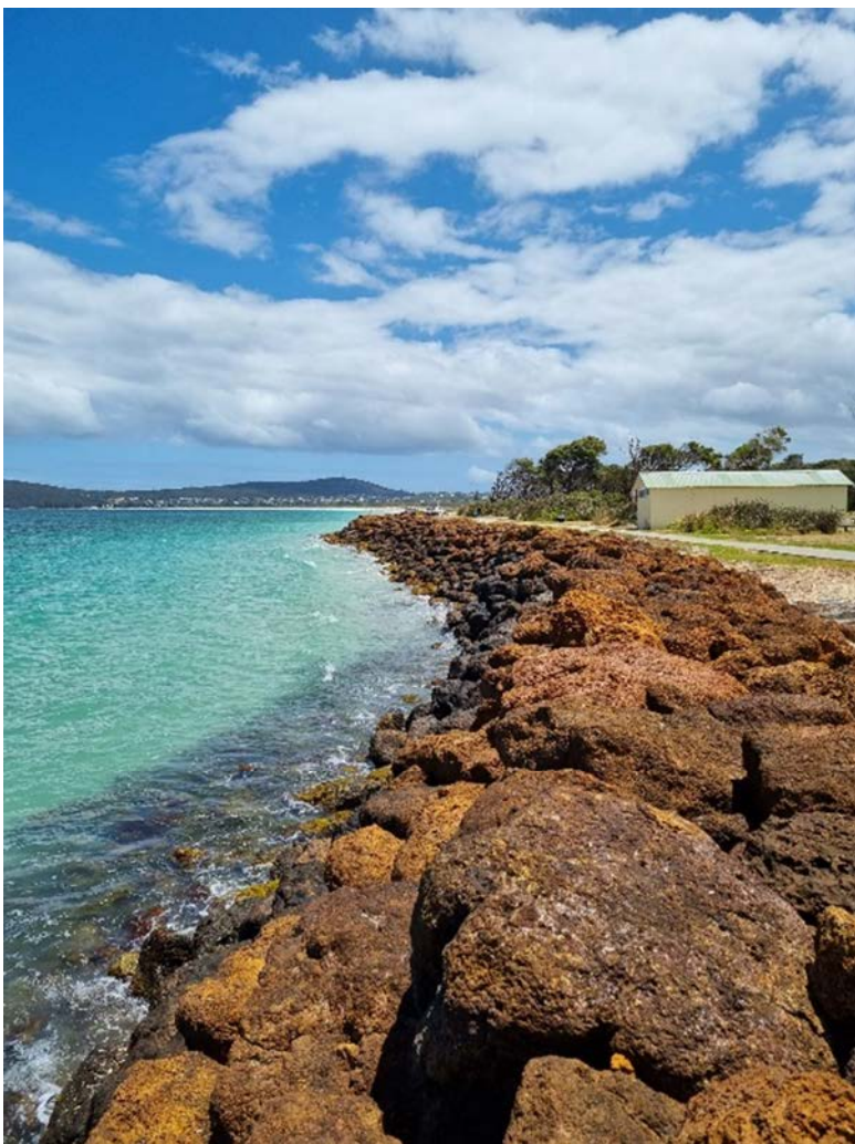
Figure 12-17: Seawall extending west (+700m) taken during site visit 5 December 2024.
