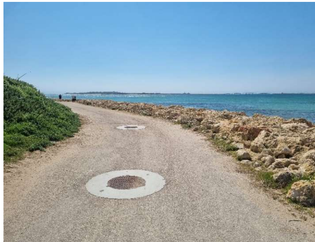
Figure 9-6: Carpark end of DBCA revetment (+3100m) taken facing west during site visit 18 September 2024.
