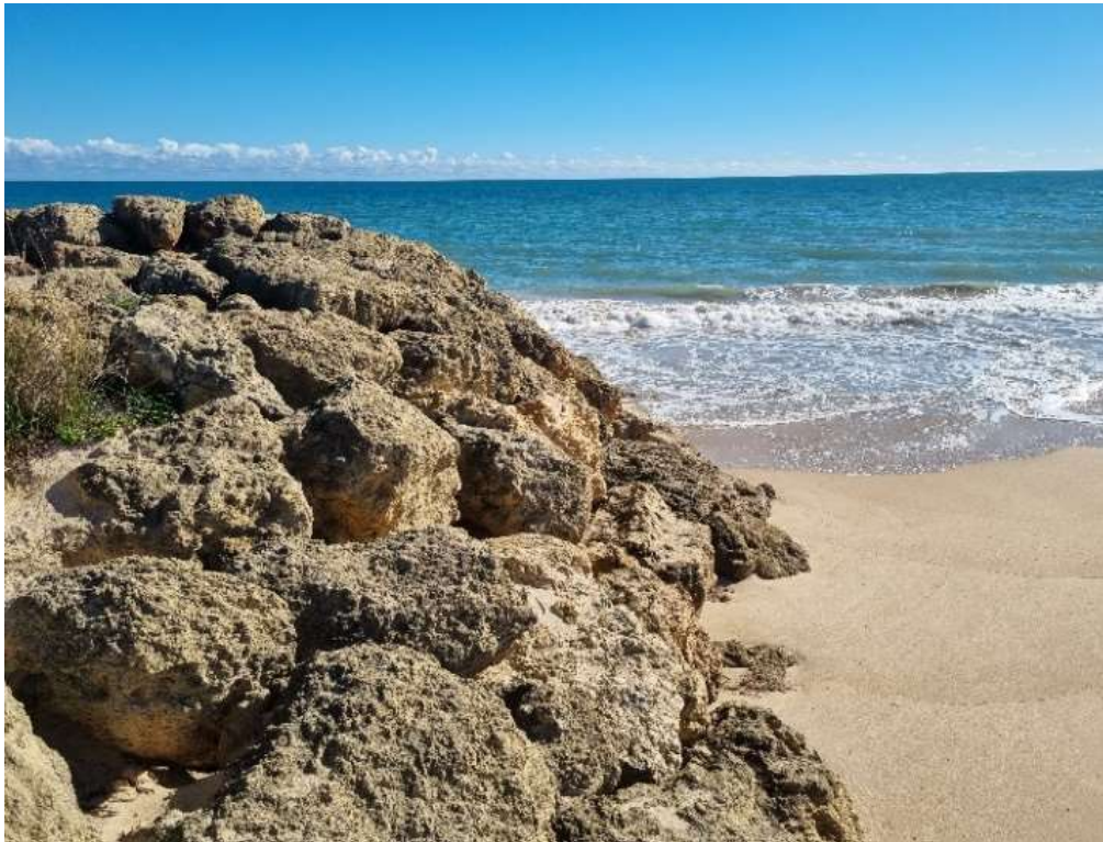
Figure 10-9: Groyne 5 (San Remo) in good condition. Taken during site visit 1 July 2024.
