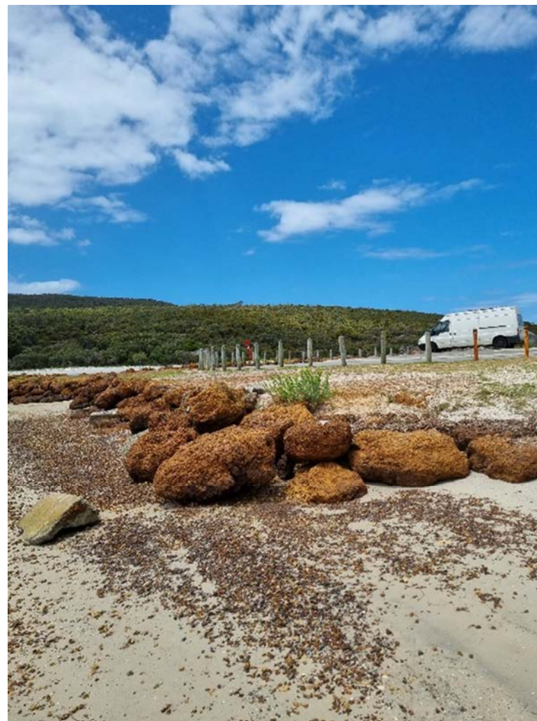
Figure 12-4: Northern seawall end, taken facing east during site visit 5 December 2024
