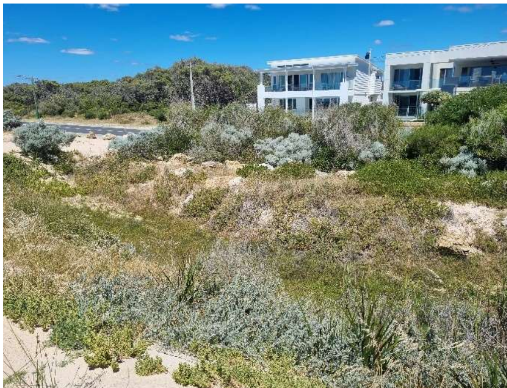
Figure 11-15: informal seawall behind primary dune (+500m), taken during site visit 27 November 2024.
