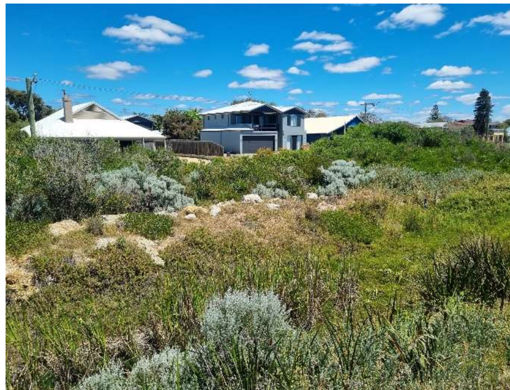
Figure 11-16: Buried informal seawall behind primary dune (+500m), taken during site visit 27 November 2024.
