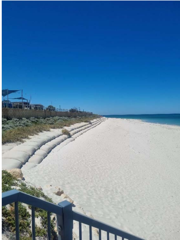
Figure 4-3: Photo taken south from access stairs at north end of section 2. GSC seawall, with lower tier containers buried, ~50m wide beach buffer (taken 11 December 2023)
