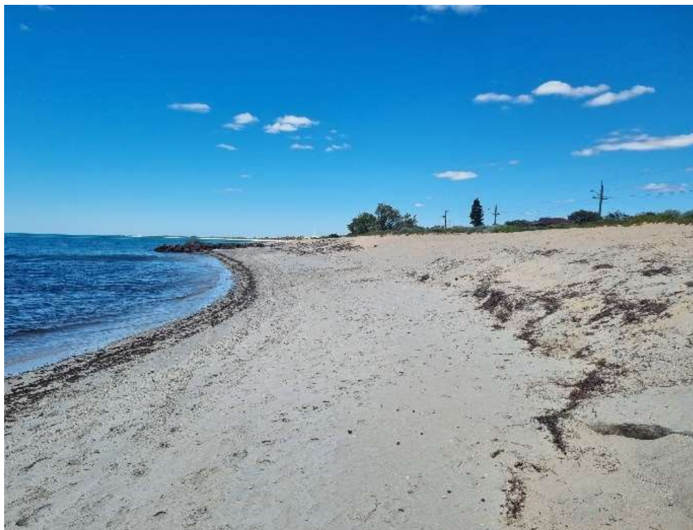
Figure 11-5: Beach compartment between Groyne 1 & 2 (+300m), beach crest consisting of recently nourished sand taken during site visit 27 November 2024.
