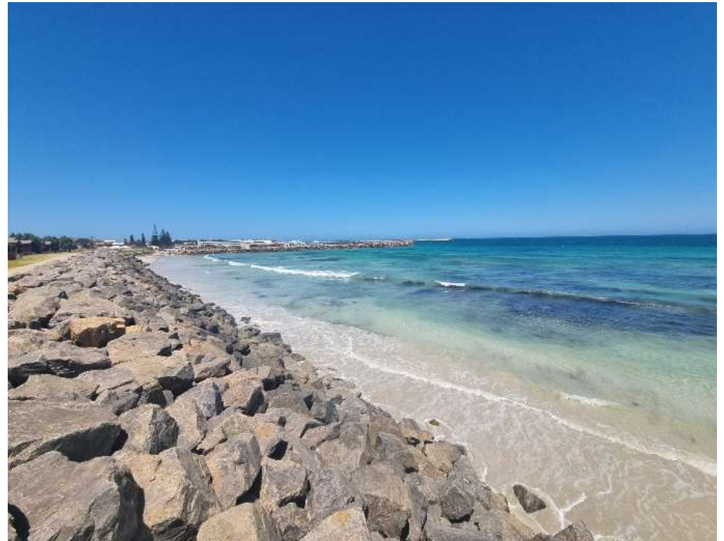
Figure 1-7: Seawall looking southwest (taken during site visit 29 January 2024)
