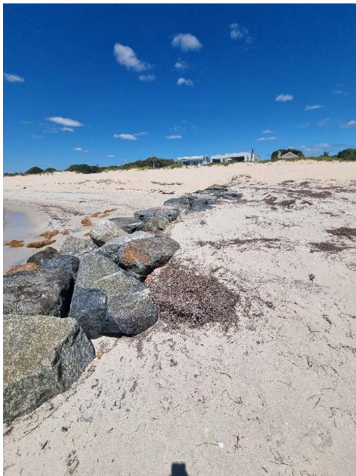
Figure 11-9: Groyne 3 (+475m), some scattered laterite immediately north, taken during site visit 27 November 2024.
