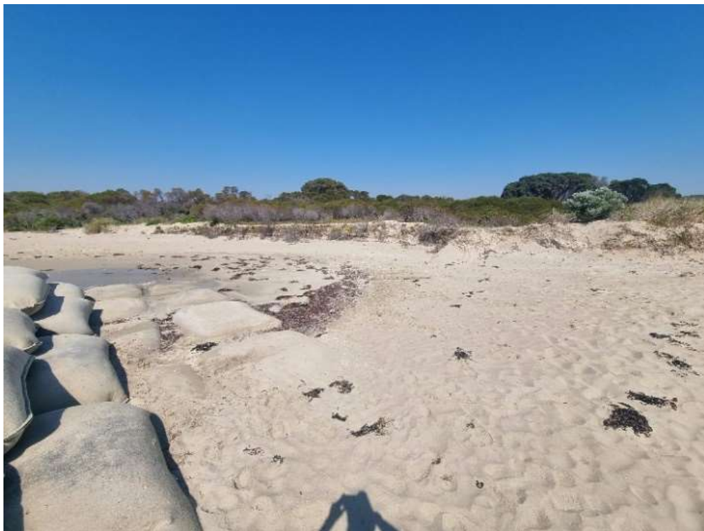
Figure 9-1: GSC groyne neck, approximate chainage +750 m. Taken during site visit 18 September 2024.
