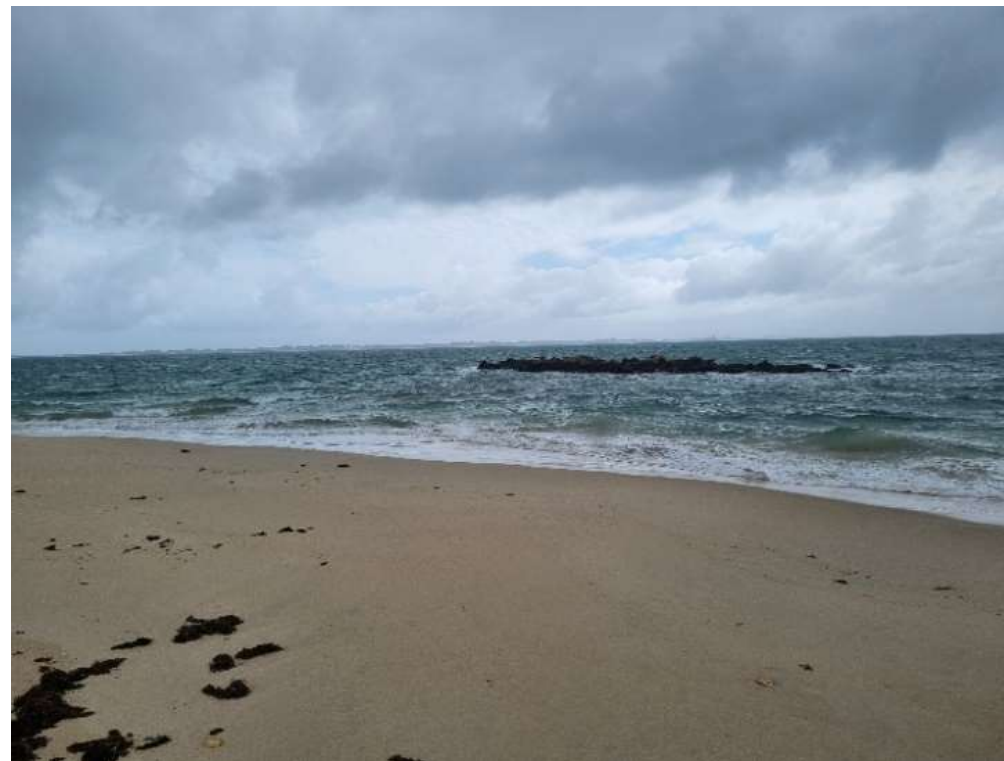
Figure 6-6: Artificial headland five (chainage +3075m) with submerged salient, taken during site visit 14 August 2024.
