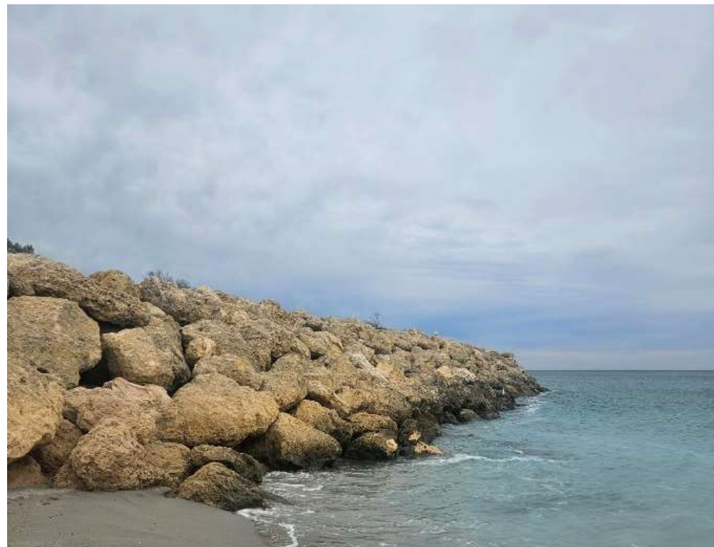
Figure 5-8: North side of Catherine Point Groyne (taken during site visit 9 May 2024)
