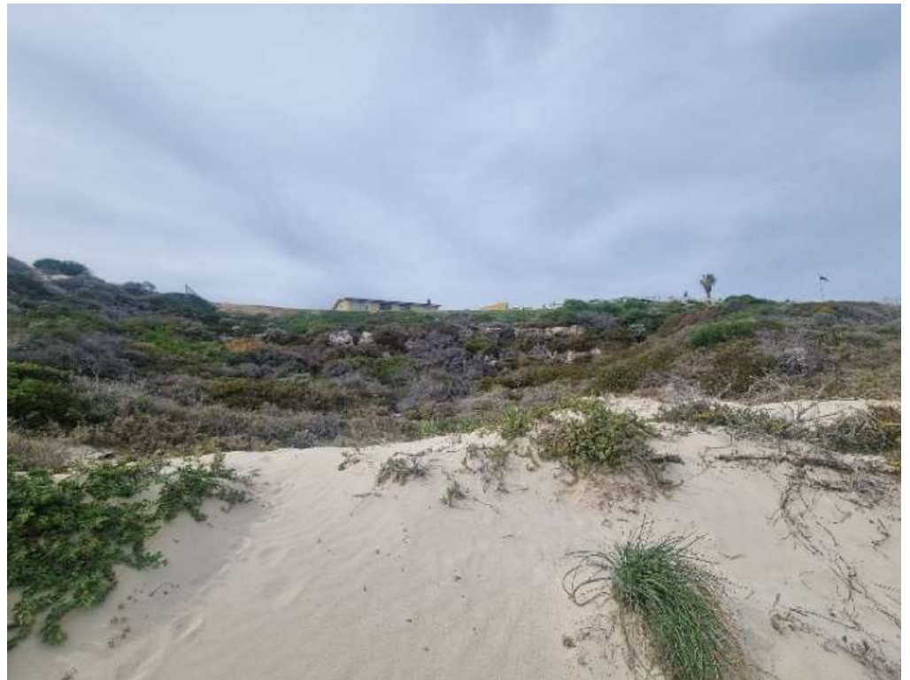
Figure 3-3: Photo taken of coastal rock protruding from dune surface (facing east) adjacent to Seabird Tavern, during site visit 20 May 2024.
