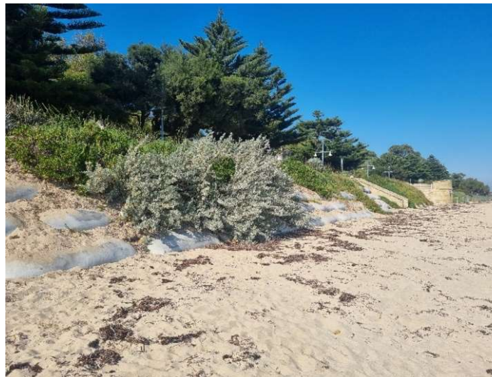
Figure 8-6: Photo taken of revegetation above Flinders Ln GSC seawall, approximate chainage +3370 m. Taken during site visit 18 September 2024.
