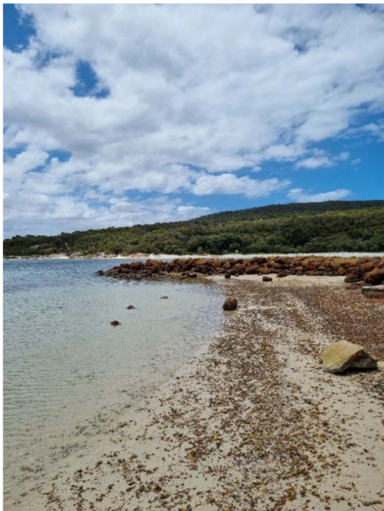
Figure 12-3: Northern groyne taken facing northeast during site visit 5 December 2024.
