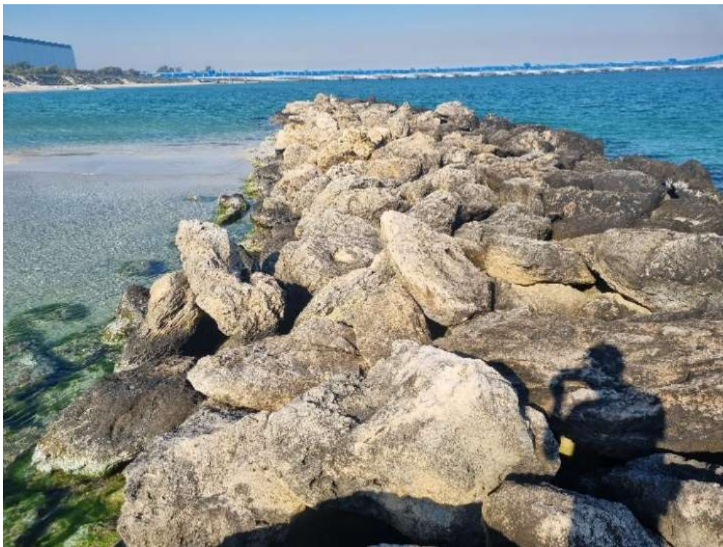
Figure 7-15: Southern artificial headland, taken from crest, during site visit 18/09/2024.
