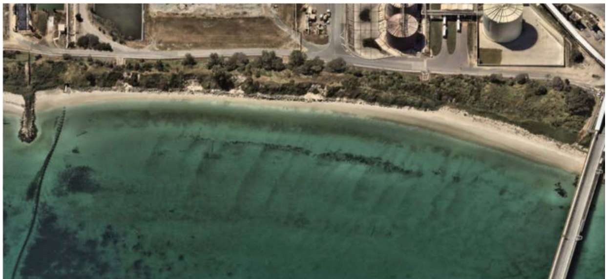
Figure 6-18: Oblique imagery of seawall adjacent to CSBP export/import pipelines to KBJ. Nearmap imagery captured 14 September 2024
