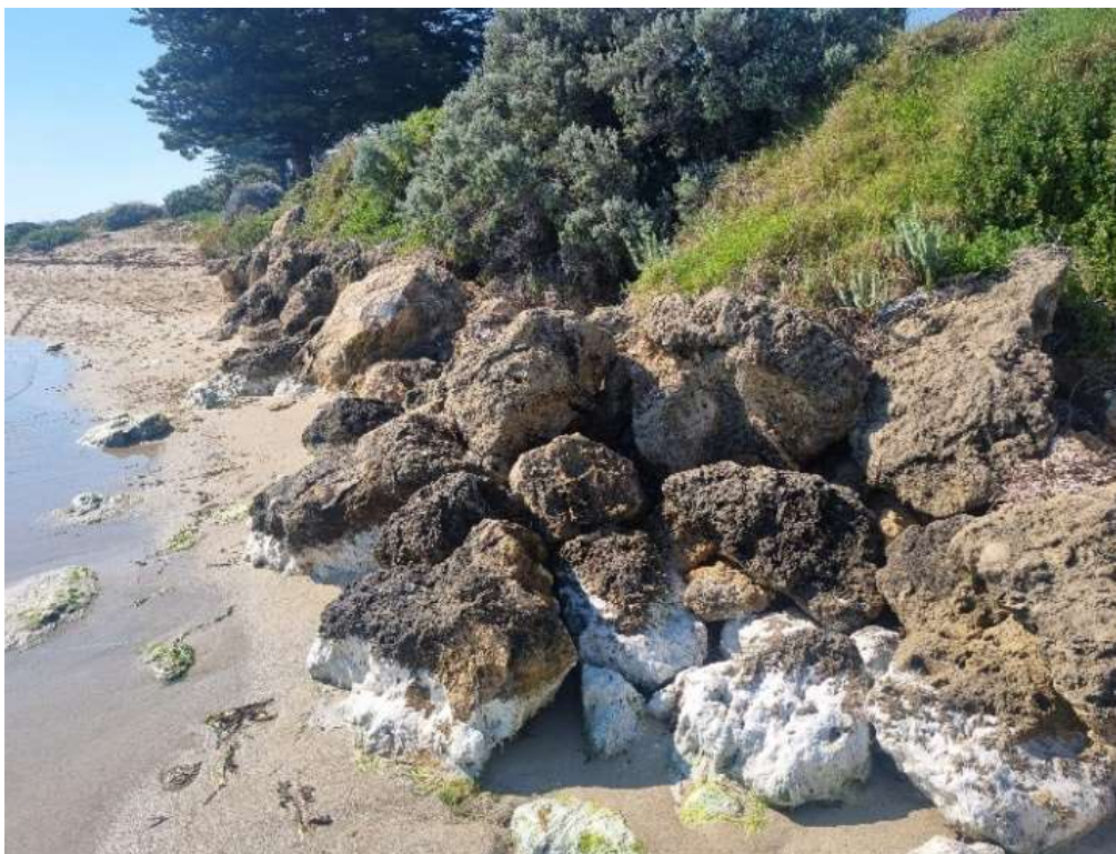
Figure 8-15: Hymus St. informal seawall (+1375m). Taken during site visit 18 September 2024.
