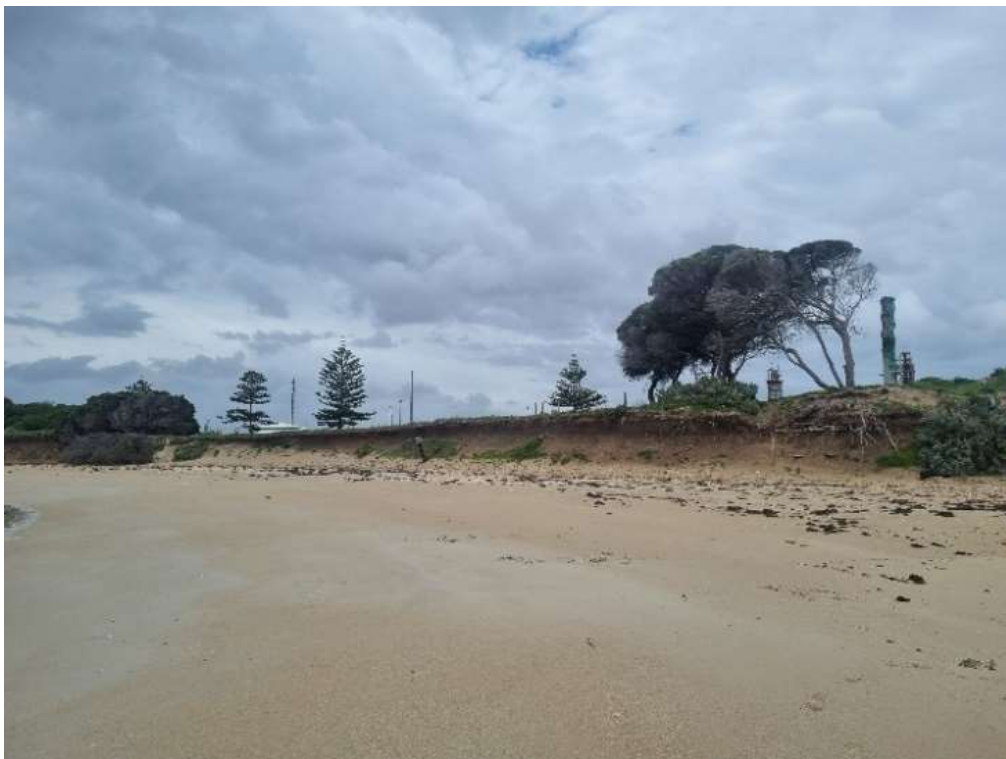
Figure 6-3: Coastal scarping and damaged ground water monitoring wells (chainage +2725m), taken during site visit 14 August 2024
