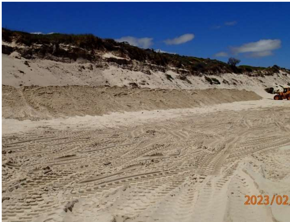
Figure 4-5: Placement of 'scraped' beach sand at base of eroding dune, taken from Groyne 4, facing south (Ellyard, 2023).
