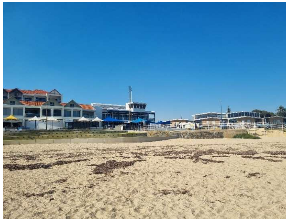
Figure 8-10: Val St. foreshore concrete retaining structures (+2925m). Taken during site visit 18 September 2024.
