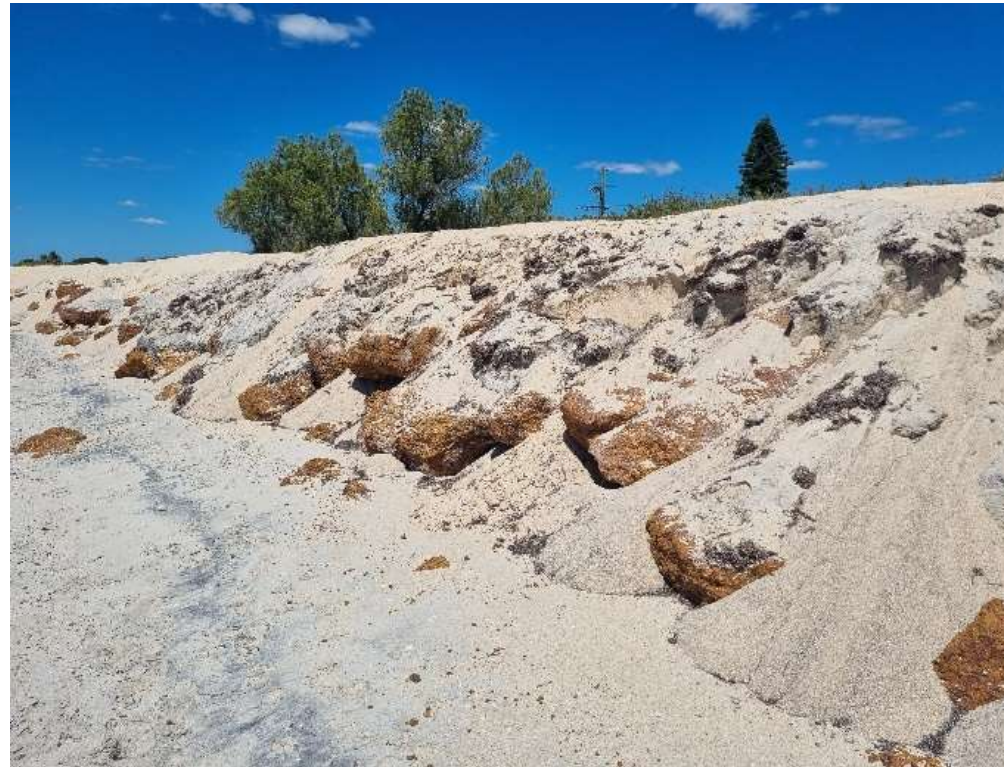
Figure 11-8: Informal seawall (+370m) taken during site visit 27 November 2024.
