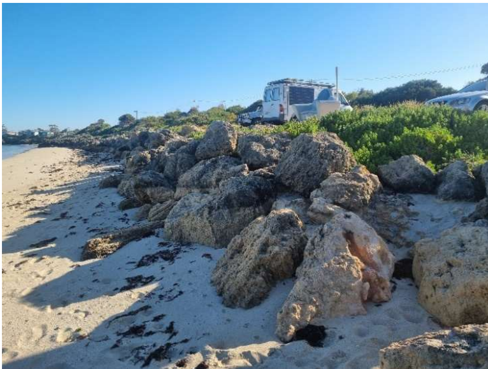
Figure 6-15: Southern end of Navy shacks rubble mound revetment, taken facing north during site visit 25 October 2024.
