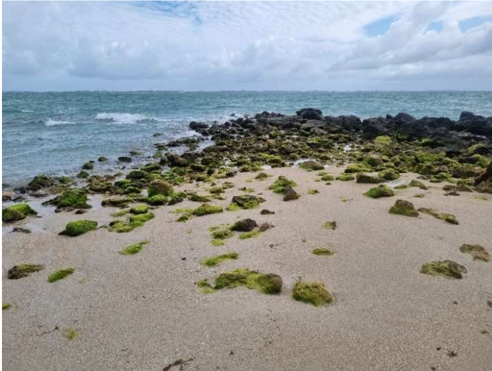
Figure 6-9: Artificial headland six (+3275m) with scattered armour, taken facing west during site visit 14 August 2024.
