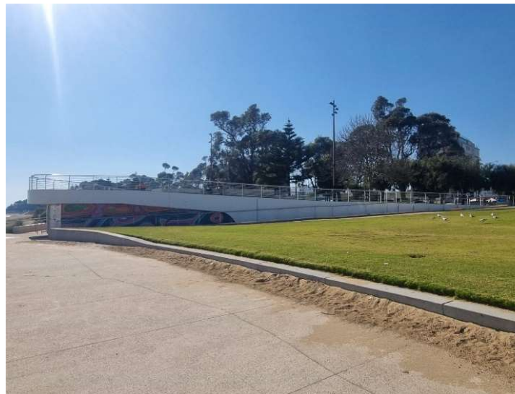
Figure 8-8: Val St. foreshore concrete retaining structures (+3000m). Taken during site visit 18 September 2024.
