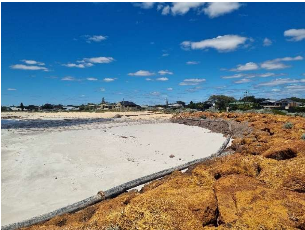
Figure 11-1: Port Geographe eastern revetment, approximate chainage +25 m. Showing dredged material being pumped onto Wonnerup beach during site visit 27 November 2024.
