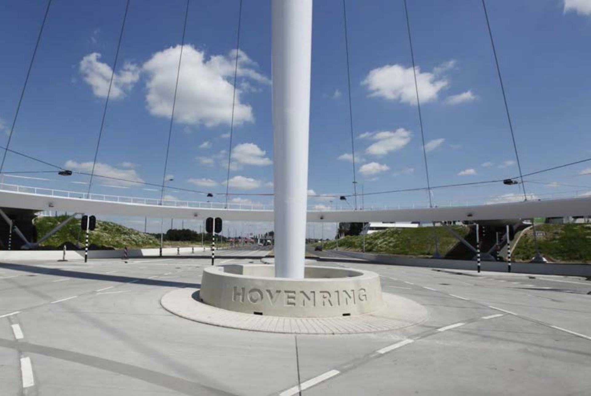
Collision Loads Concrete Barrier Pylon Foot
