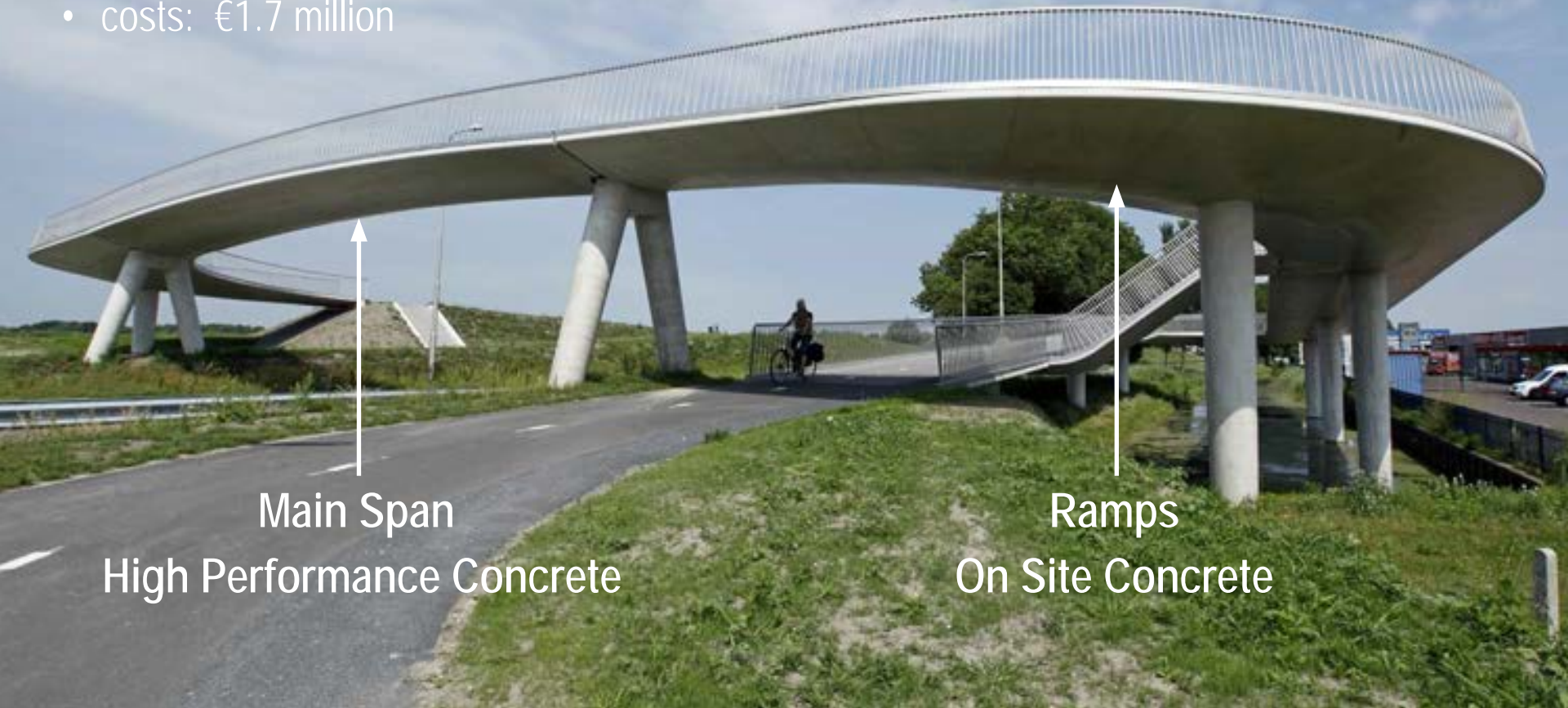
Heerhugowaard Station bridge Maintenance Free Main Span
