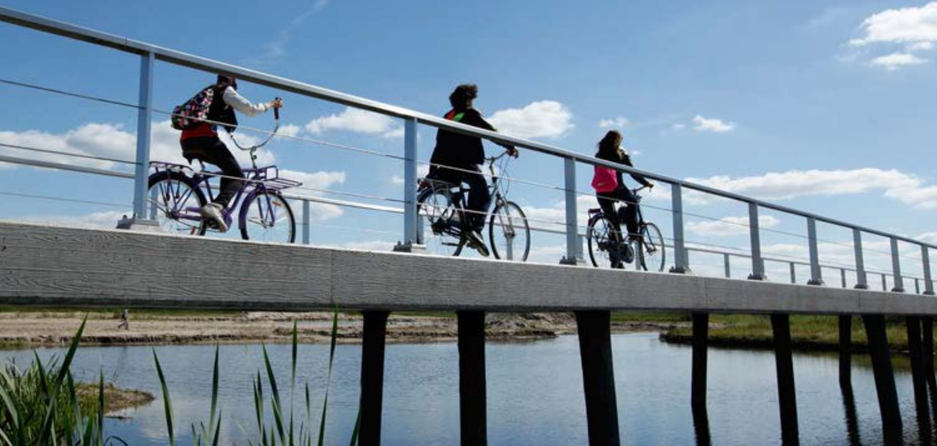
Breda Werkdonken bridge benefits from the context
