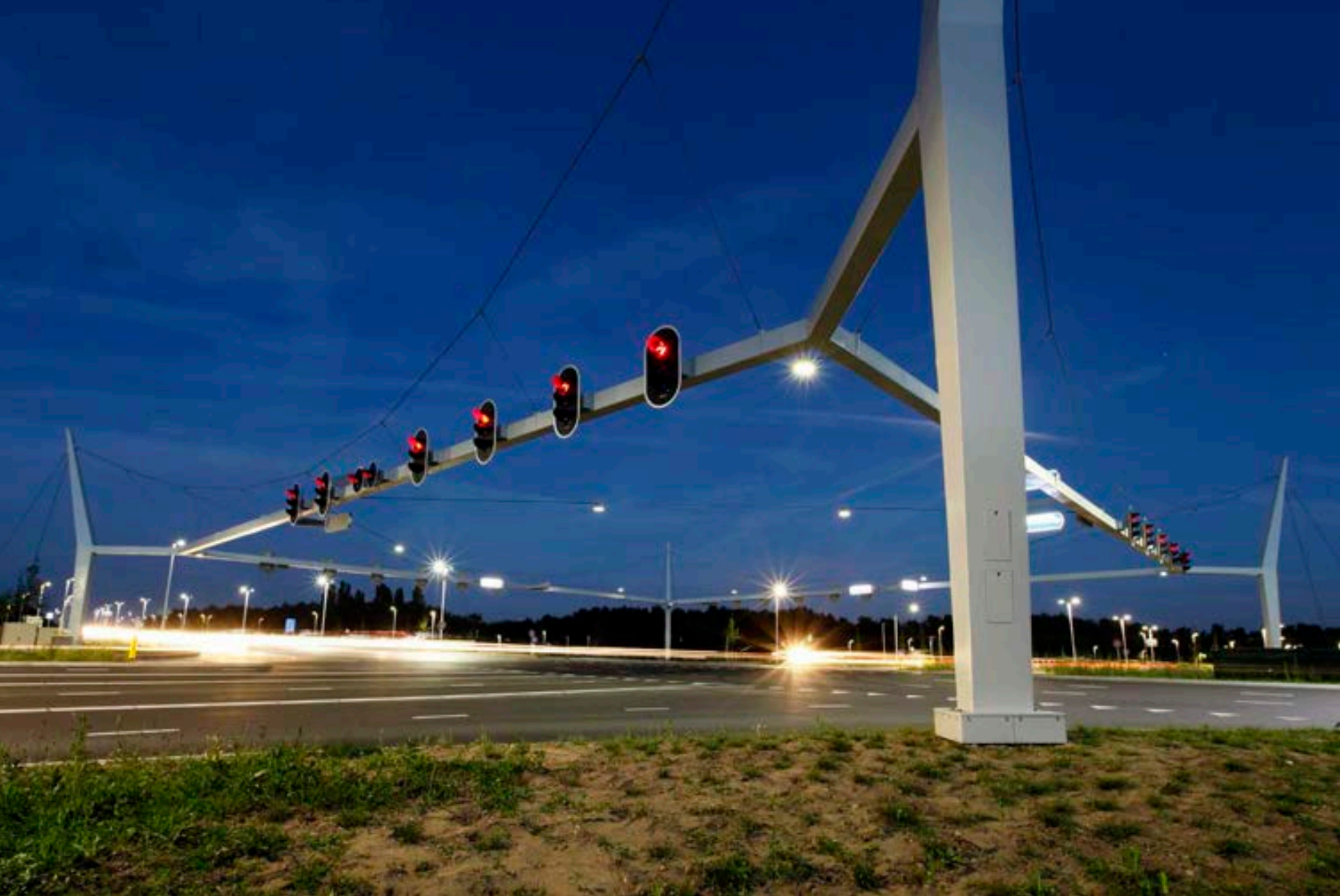
Integral Design Integration of traffic lights, lighting and signage
