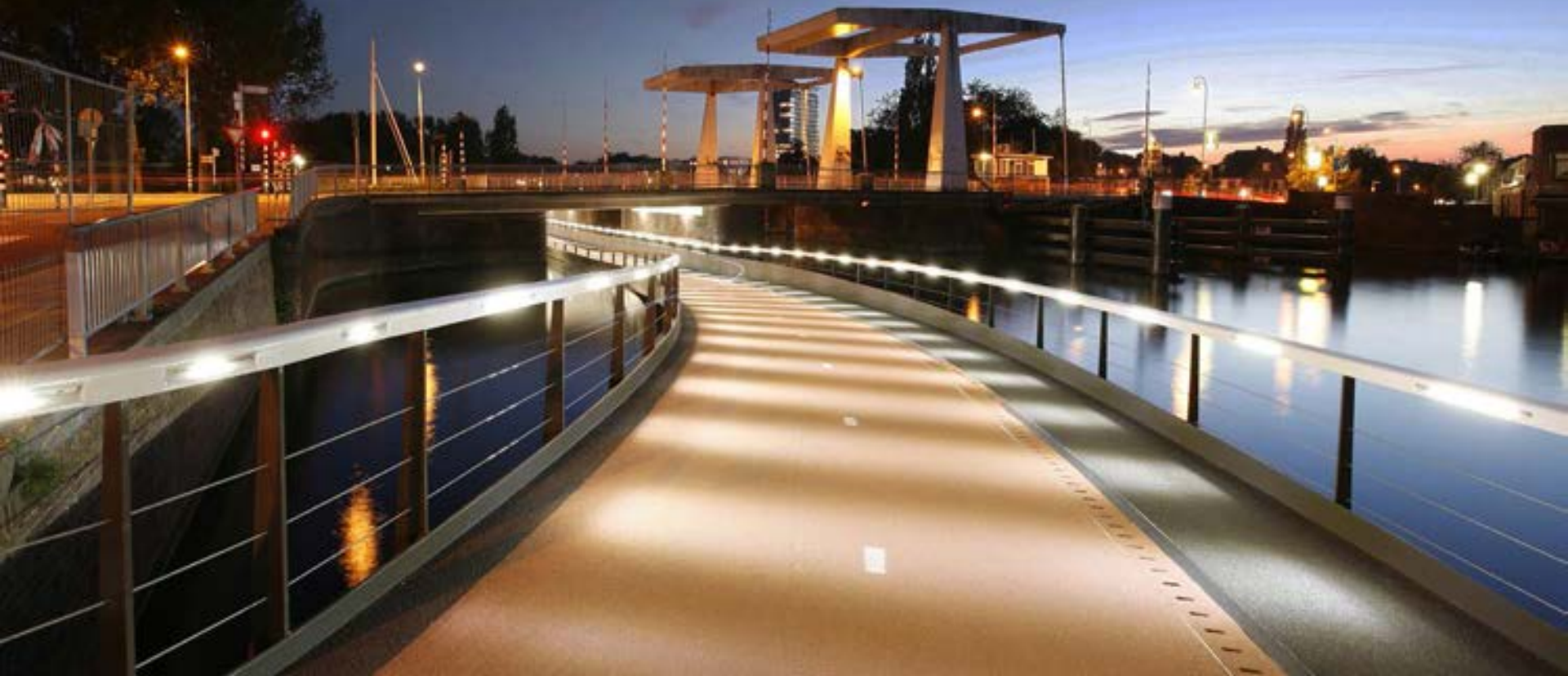
Haarlem submerged bridge Result
