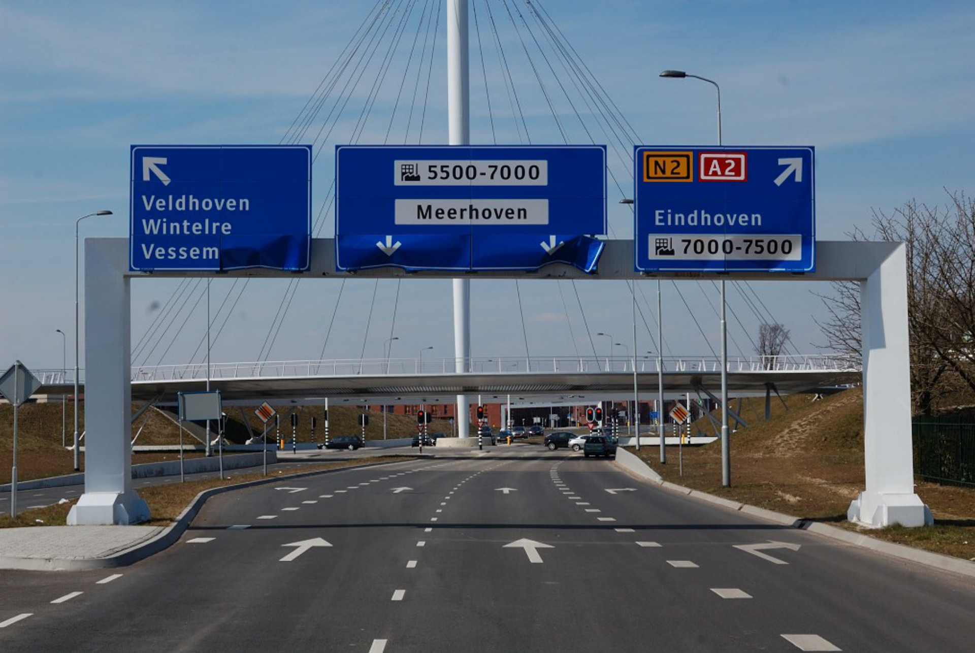
Collision Loads Anti-Collision Portals proven usefull
