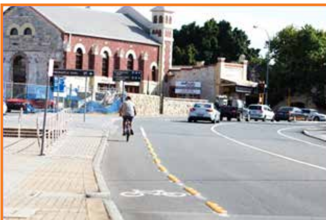
Bike lane separated with mountable plastic kerbing
