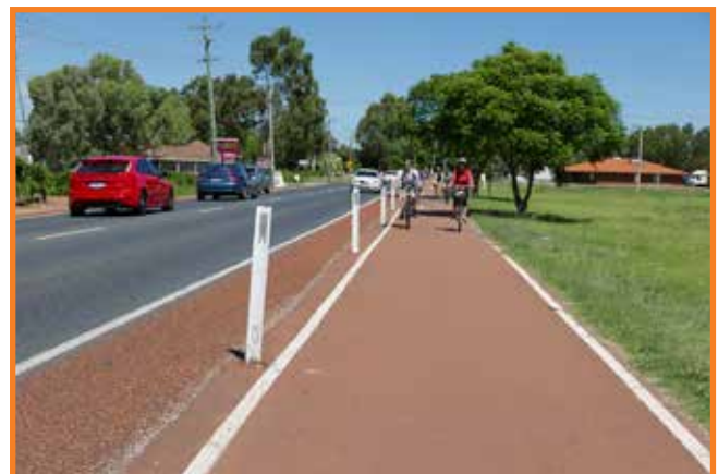
Bi-directional bike lane separated with bollards
