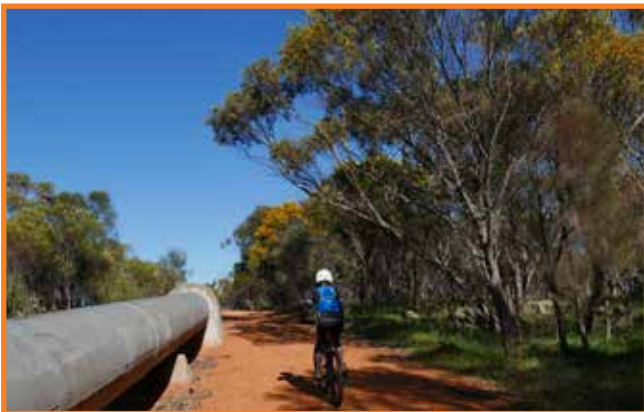
Trail within utility corridor
