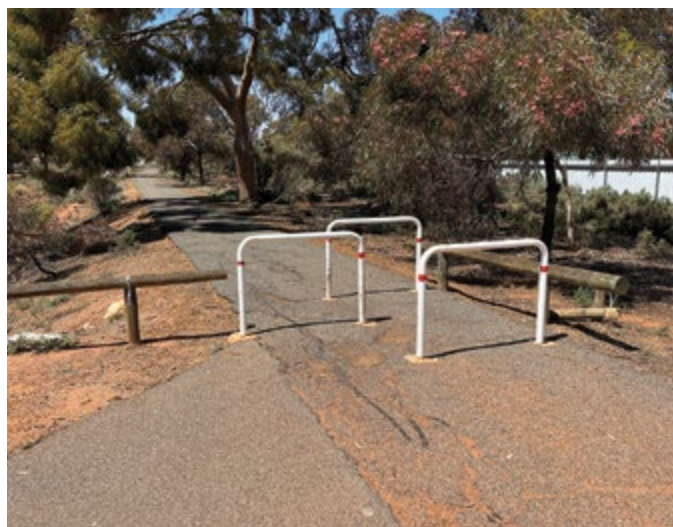
Change in path surface and width along a shared path (left) and grabrails restricting the path of travel (right). Credit: Department of Transport.
