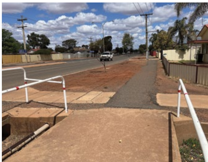
Change in path surface and width along a shared path (left) and grabrails restricting the path of travel (right). Credit: Department of Transport.
