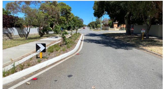
Figure 8: Lane narrowing using formalised parking
