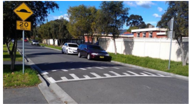
Figure 5: Road hump – Watts profile
