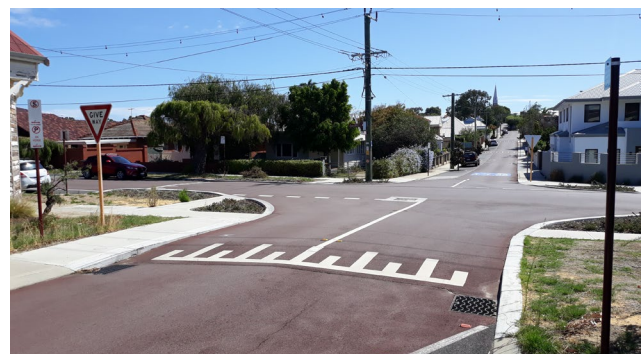
Figure 4: Raised pavement – all approaches
