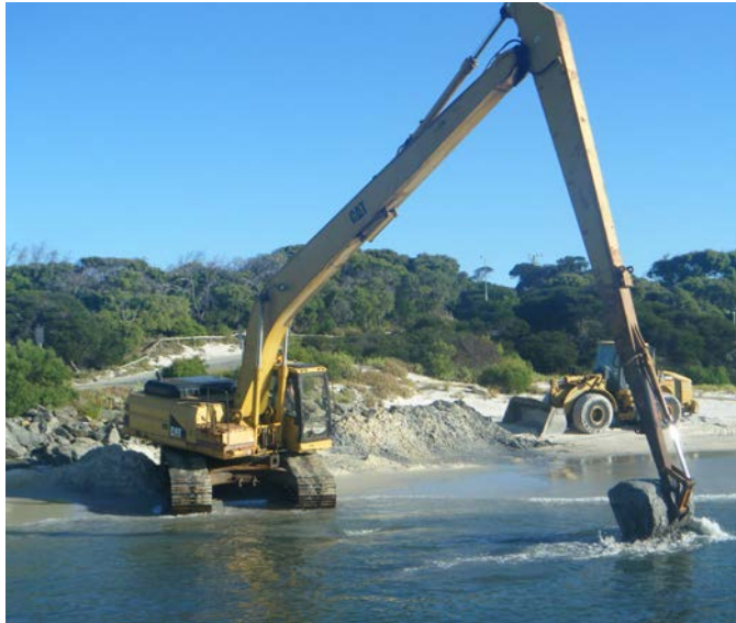
Excavation from shore – Bremer Bay 2010
