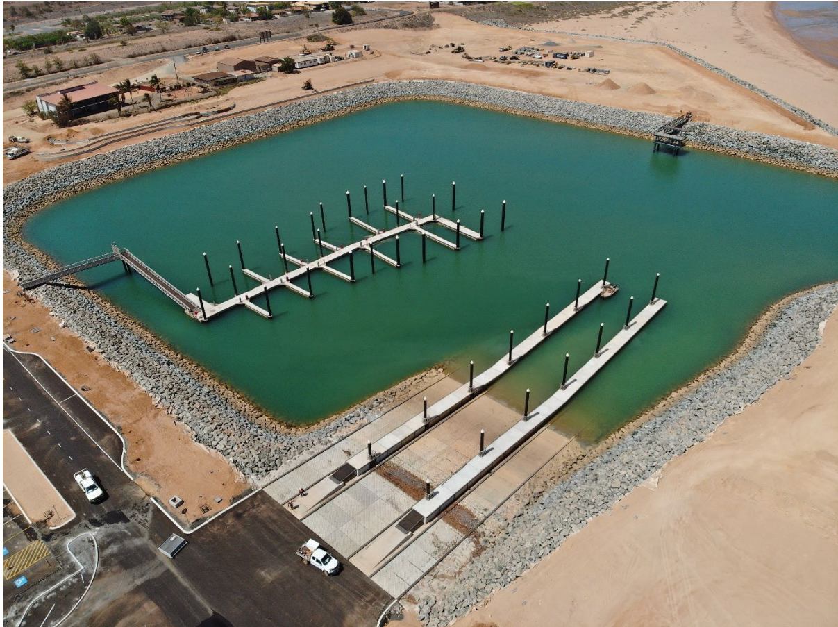
Figure 2: Aerial view of Spoilbank Marina Boat Pens
