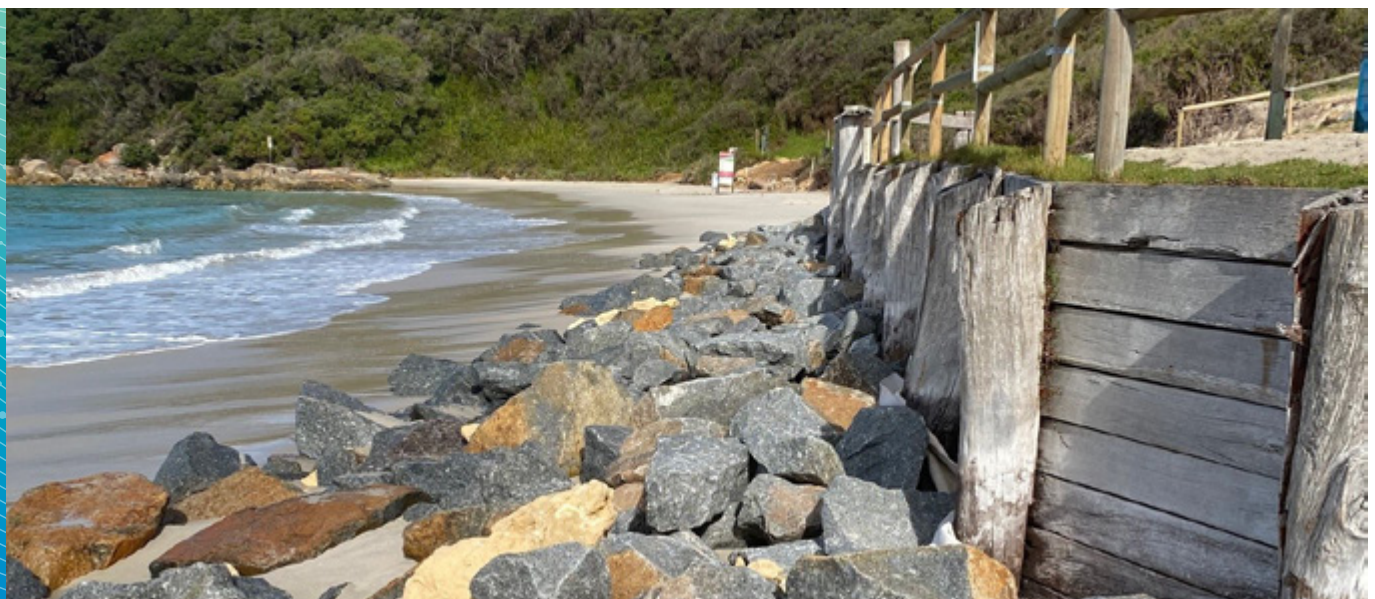
Retaining wall Ocean Beach, Shire of Denmark
