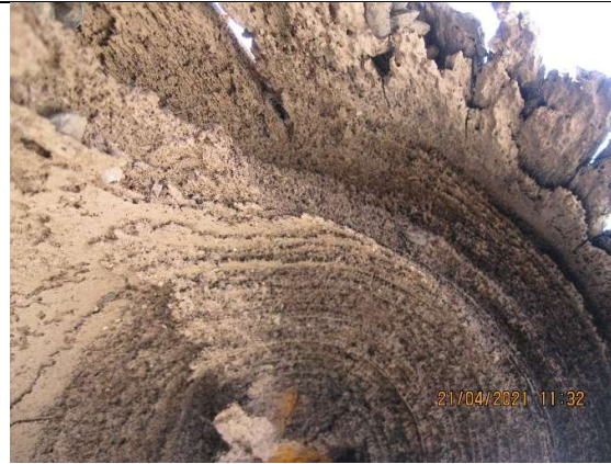
Photo 32: End view of pile at top of photo (Photo 31)
