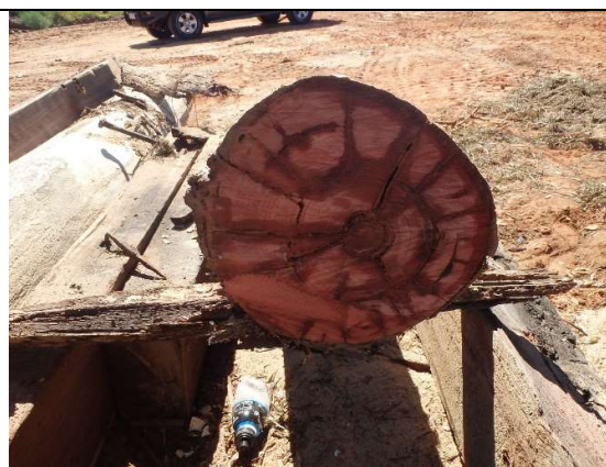
Photo 28: Further section above rot area confirming that Teredo not present
