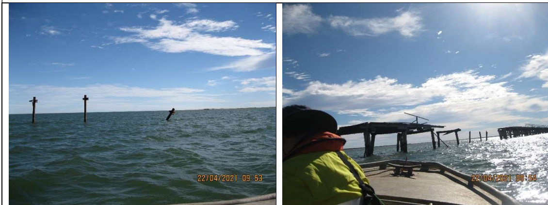
Photo 8: Jetty Approach between Piers 186 and 218
