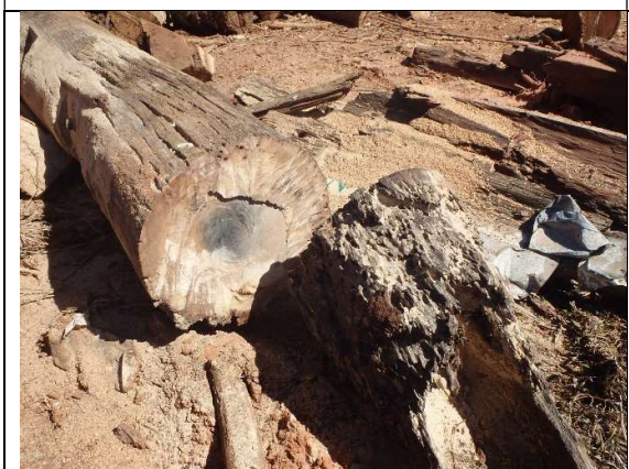
Photo 29: Salvaged pile cut just above necked area (MSL) – no evidence of Teredo
