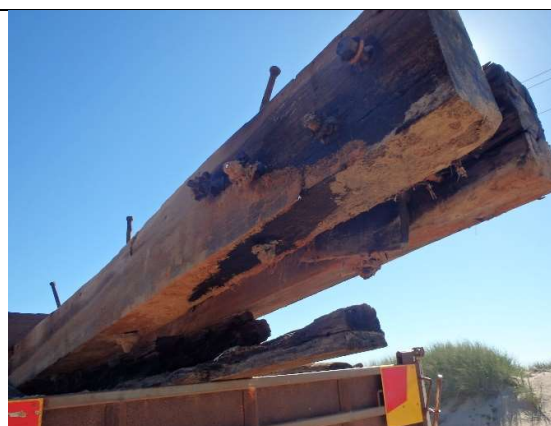
Photo 30: Salvaged Crosshead showing bolts in place where corbels were secured
