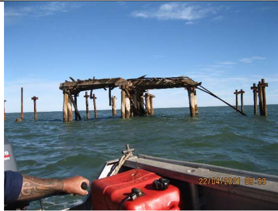
Photo 2: Portion of jetty head - note steel piles remaining.
