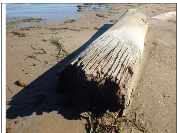
Photo 25: Typical pile showing break at waterline due to rot and Linnoria attack.
