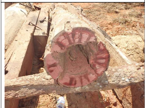
Photo 27: Salvaged pile cut just above necked area where pile snapped showing internal rot
