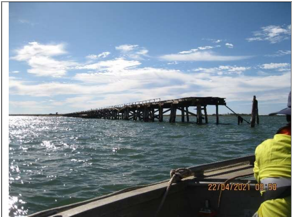
Photo 10: Approach jetty Shallow area - Piers 70 to 186
