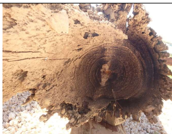
Photo 26: View inside snapped pile
