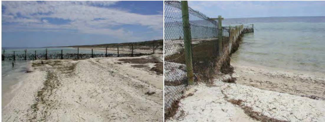
Figure 6-4: Sediment and Wrack Capture at Peron Fence 25 October 2006 (Source: Damara WA 2006e)
