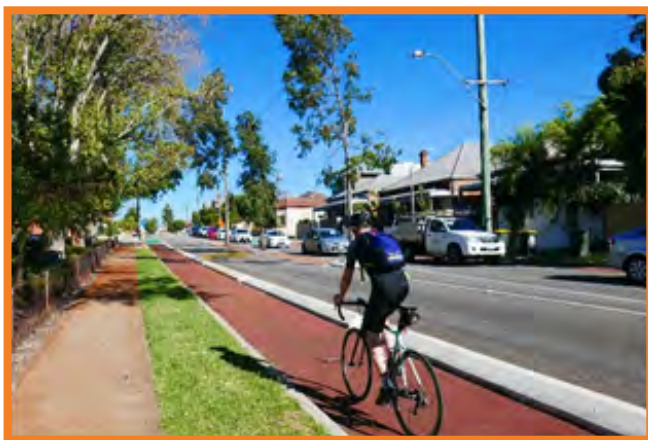
Bike lane protected with concrete kerb
