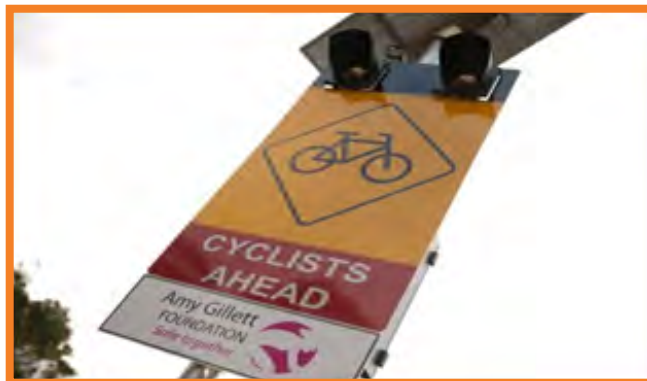
Dynamic flashing warning lights (Victoria)
