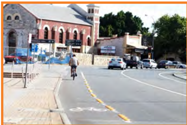
Bike lane separated with mountable plastic kerbing
