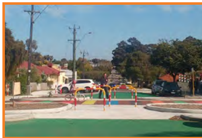
Mid-block road closure
