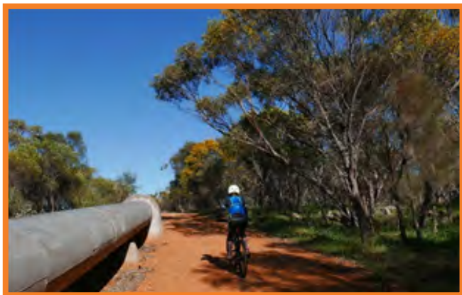
Trail within utility corridor
