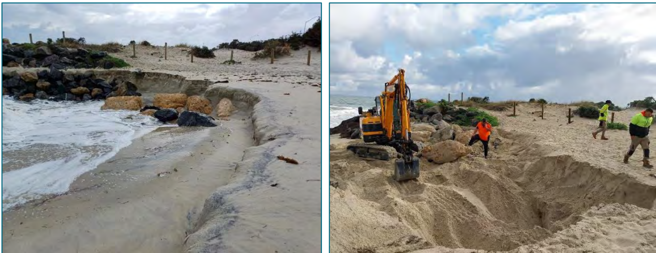
Figure 37: Port Beach in July 2024 with seawall flank erosion (left) and boulder relocation (right) following winter storms (sourced from City of Fremantle survey).
