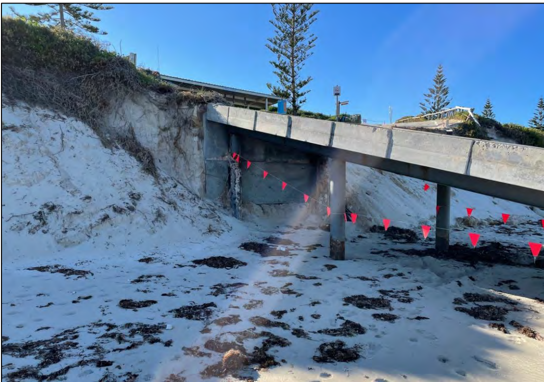
Figure 27: Erosion north of seabird revetment in winter 2021 showing closed off access at both the stairs (top) and caravan park ramp (bottom) (sourced from DoT 2022).
