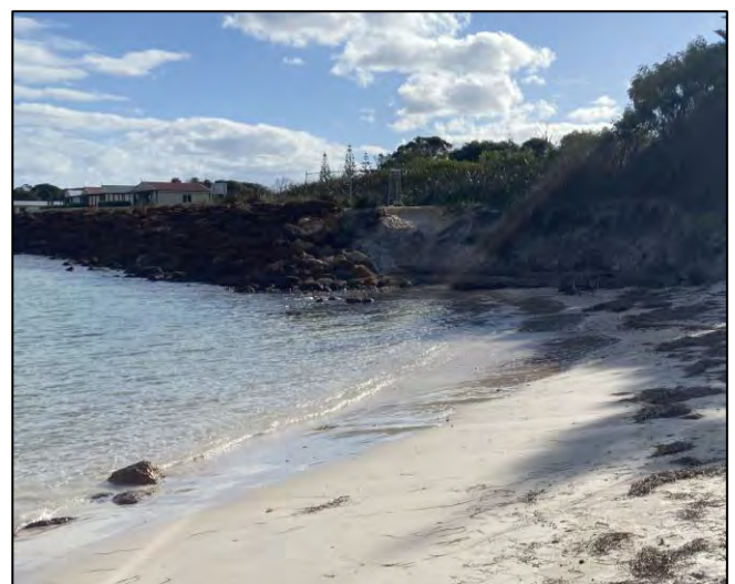
Figure 59: Emu Pt, Albany Hotspot in 2016 (left) and 2024 (right) on the flanked eastern section of revetment. 30m of shoreline recession and destroyed beach access is evident.
