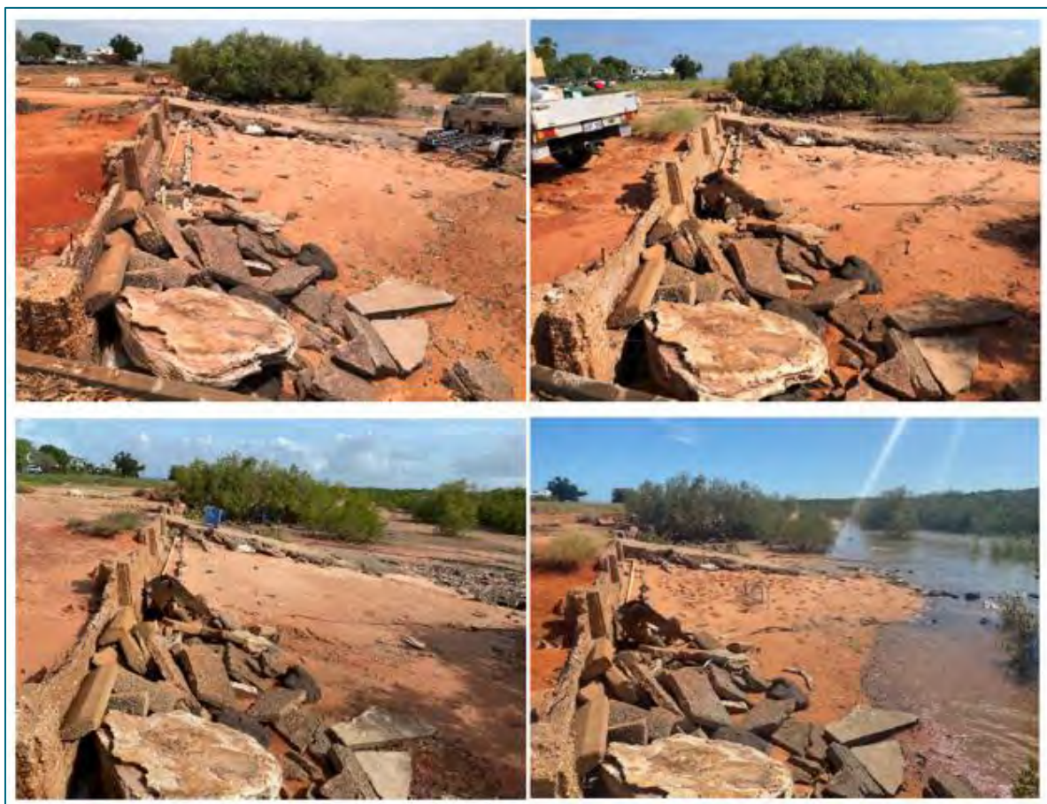
Figure 11: Example of dilapidated protection structures at China Town, Broome hotspot; images taken are from Dec 2018 (top left), Feb 2019 (top right), Jan 2020 (bottom left), and Apr 2020 (bottom right) (sourced from Shire of Broome survey).
