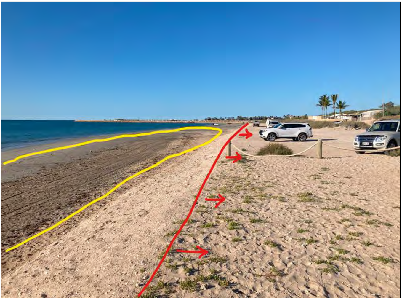
Figure 14: Hotspot at Warne St & Yacht Club Exmouth (date unknown) showing sand build up from bypassing (red area) and dredge spoil (yellow area) (sourced from Shire of Exmouth survey).
