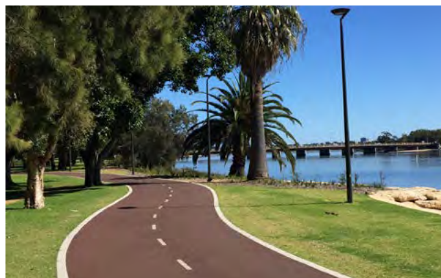
Figure 11.3 Path “deviation” around established tree.
