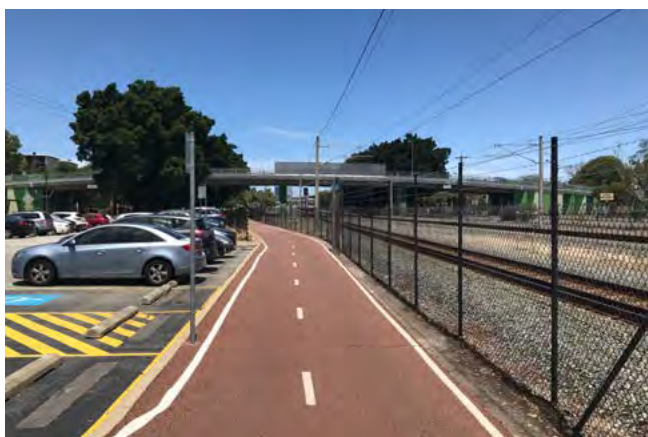
Figure 9.5 Edge line example.
