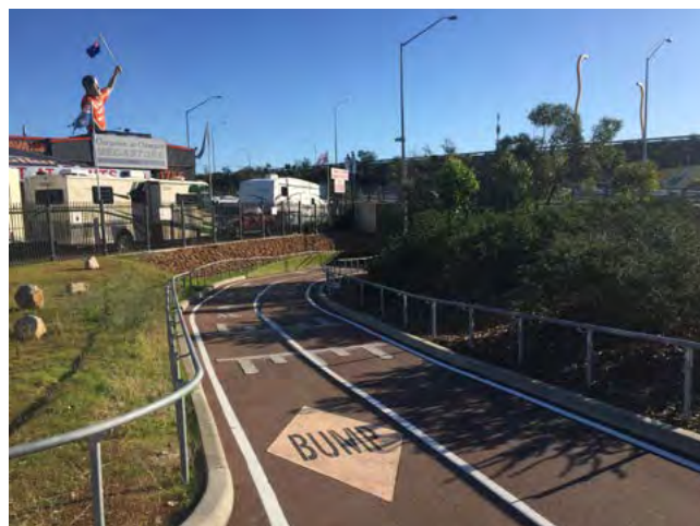
Figure 3.8 Examples of ‘BUMP’ and piano key pavement markings.
