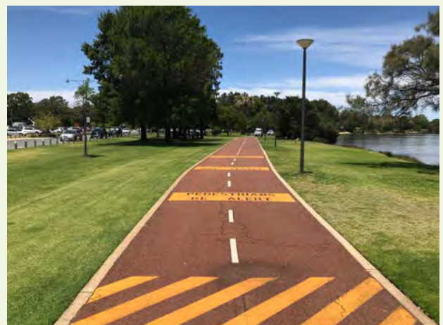
Figure 10.6 Transition ramps from Shared paths to on-road cycle facilities.
