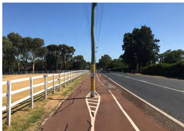
Figure 10.4 Obstruction treated as bollard.
