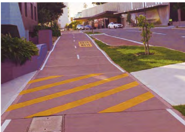
Figure 9.10 Yellow diagonal markings used to designate area where vehicles cross path.
