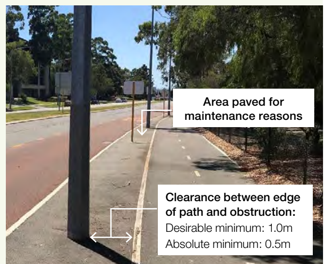
A minimum clearance of 0.5m is required between the edge of path and any obstruction e.g. lamp and signposts.
