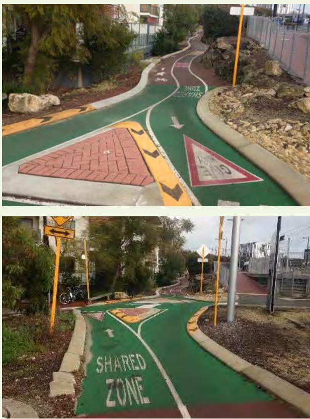
Figure 10.9 Example of path deflection pedestrian crossing (note the extensive use of warning signage and pavement markings to further reinforce).
