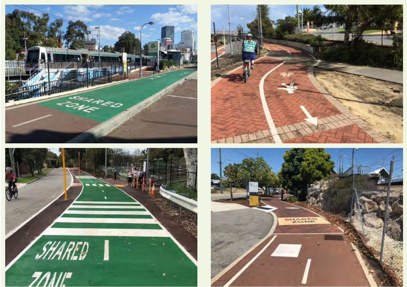
Figure 10.8 Examples of alternative pavement materials & colours used in areas with high pedestrian activity.
