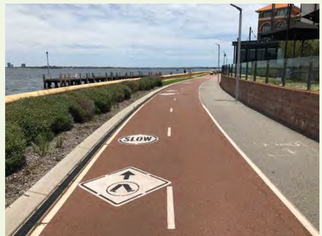
Figure 10.7 Examples of pavement markings used to promote slower cycling in areas of high pedestrian activity.
