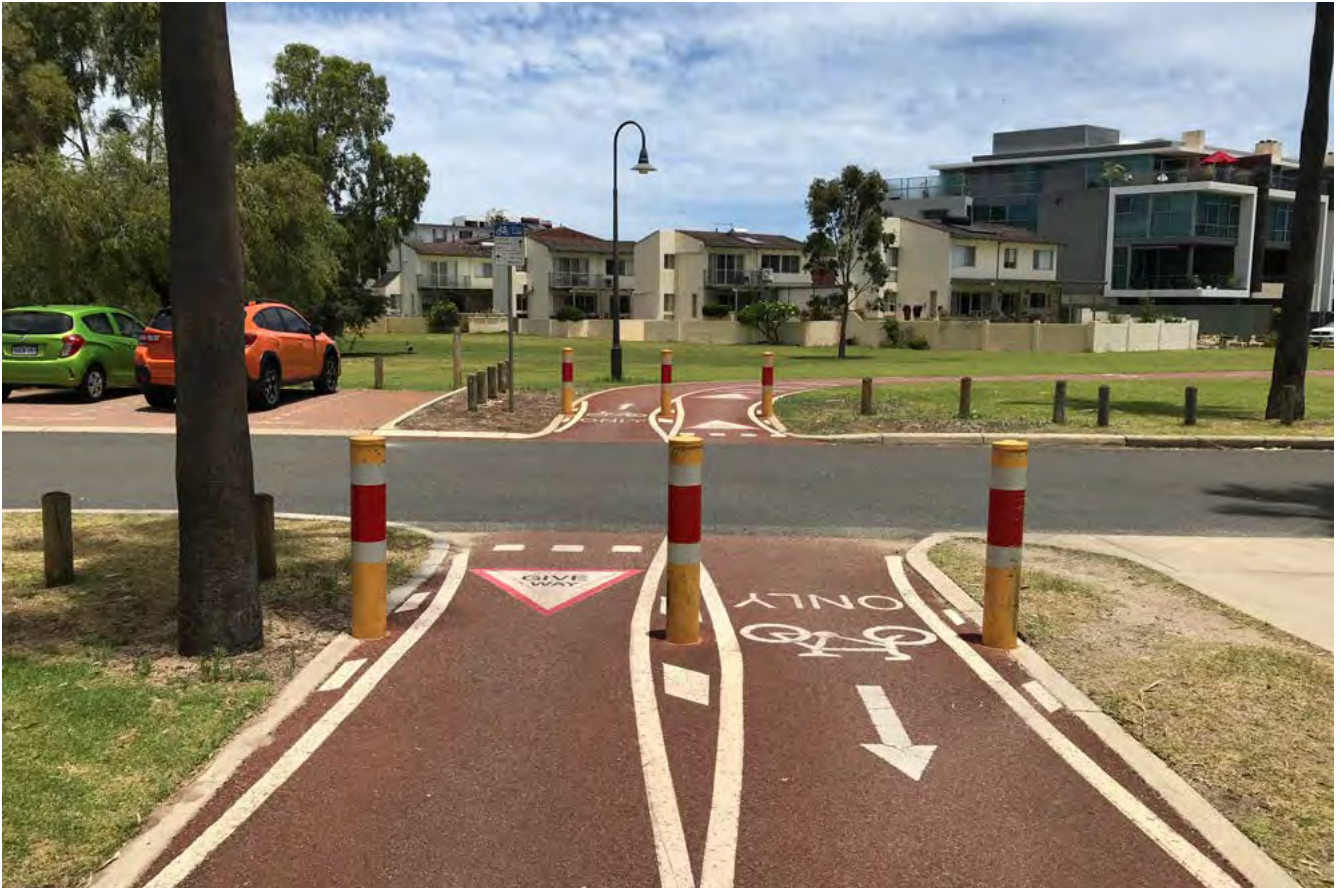
Figure 10.14 Preferred entry bollard treatment for preventing unauthorised vehicle access.
