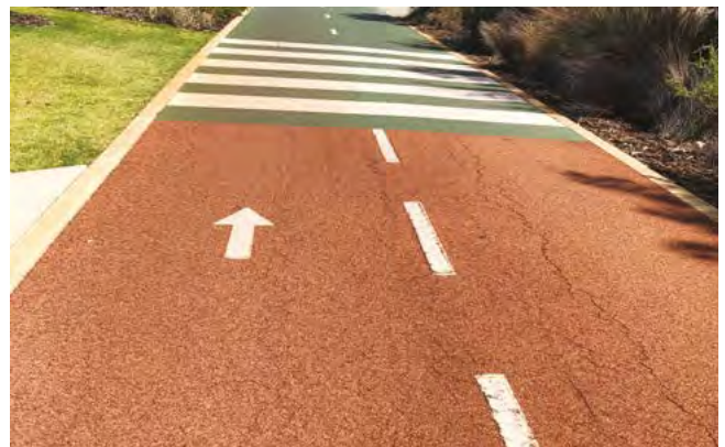
Figure 10.11 Rumble strip treatment using thermoplastic line marking.
