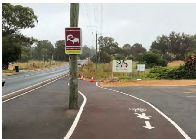
Figure 10.3 Path deviation around obstruction.
