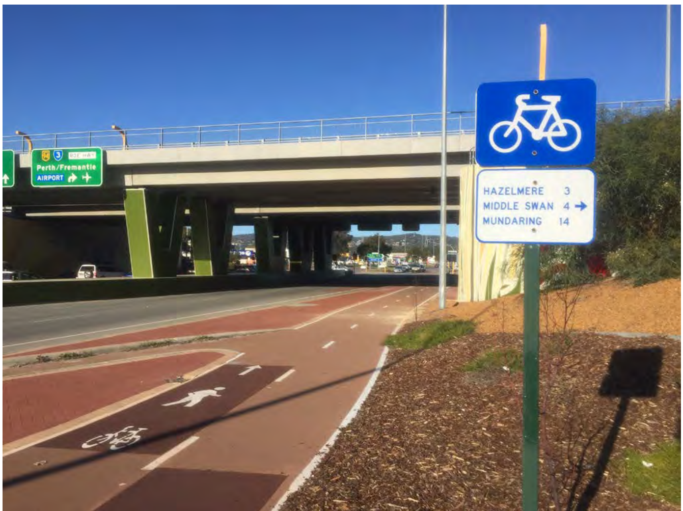
Figure 9.1 Directional signage installed outside of the path envelope.
