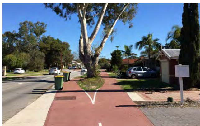
Figure 11.4 Path “split” around established tree.
