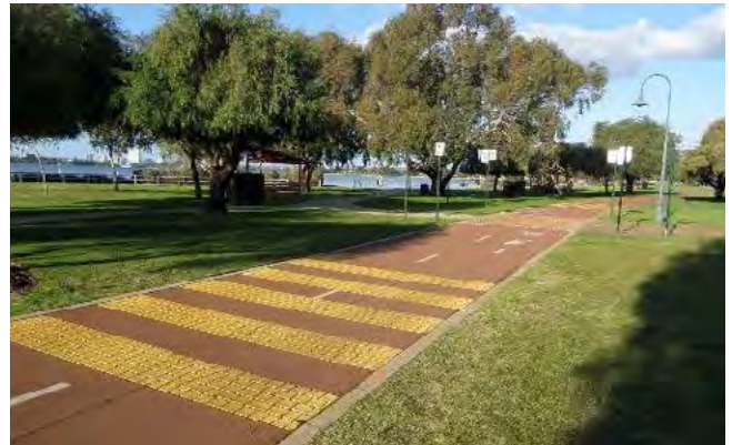
Figure 10.10 Rumble strip treatment using brick pavers.
