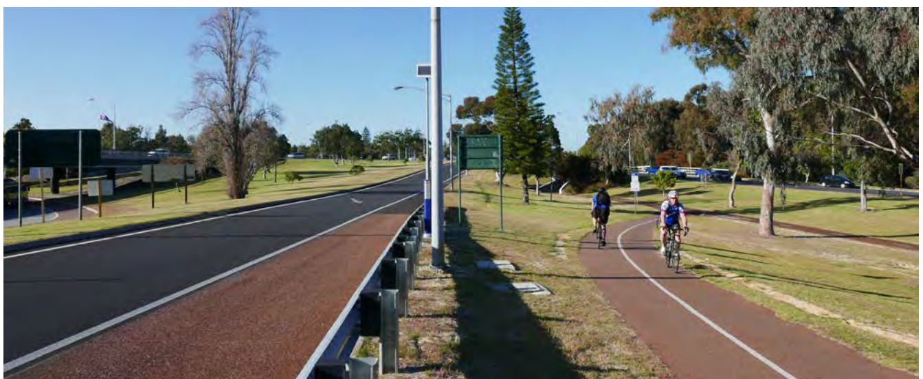
Figure 7.2 Safety barrier separating shared path from high-speed road.
