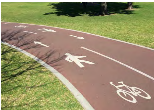
Figure 5.1 Red asphalt is the preferred surface treatment for all “cycling-focussed” paths in Western Australia.
