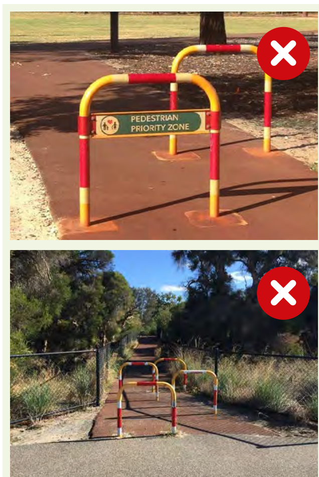
Figure 10.12 U-rails not supported as a conflict management treatment on shared paths.
