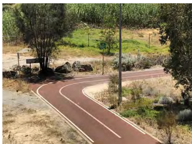
Figure 3.6 Sharp 90° bends on paths should be avoided, as bike riders will not be able to remain on the correct side of the path as they corner.
