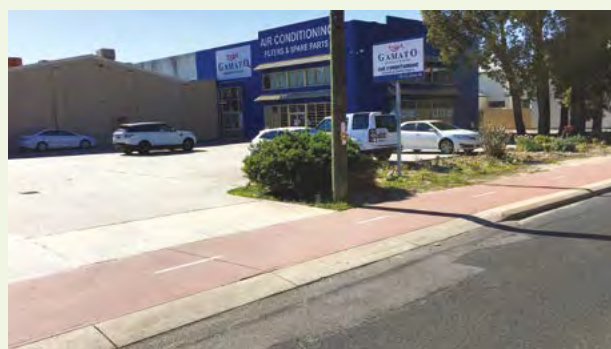
Mountable kerb used in driveway location.
