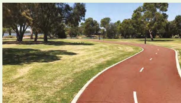
Flush edge kerb used to provide a boundary between path and landscaping.
