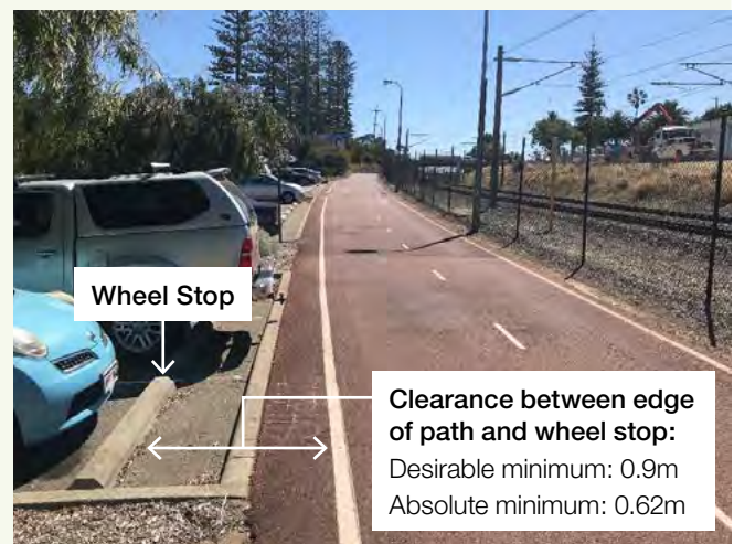
Wheel stops used to prevent parked vehicles from overhanging onto shared path.
