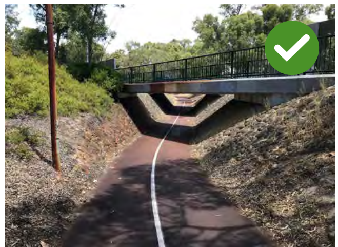
Figure 3.14 Example of clear sightlines below an overhead obstruction.
