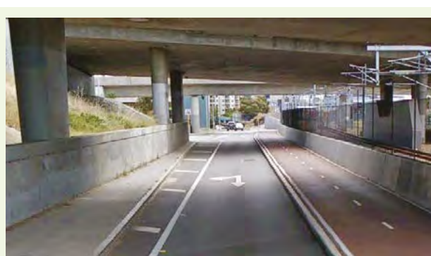
Barrier kerb used to separate path users from traffic.
