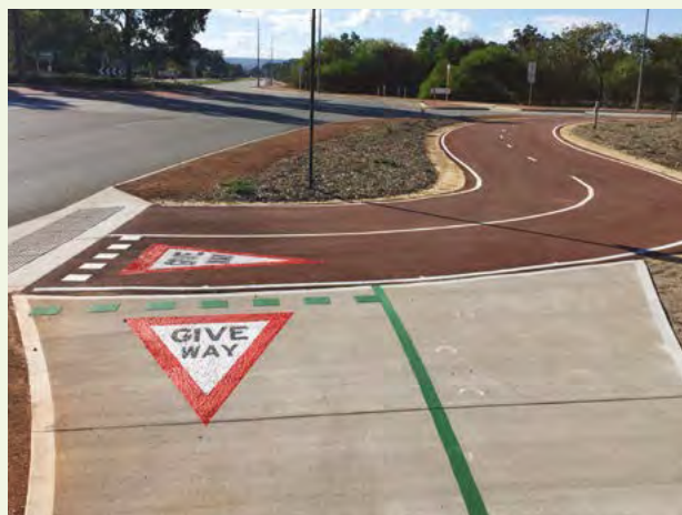
Figure 9.7 Give Way line examples.
