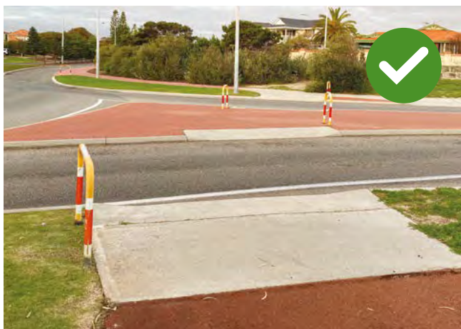
Figure 4.12 Holding Rails – must be placed on the left side of the path within easy reach of rider.
