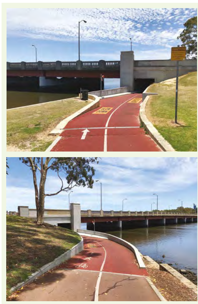
Figure 3.2 Where space constraints result in substandard geometry, advisory measures are recommended to encourage appropriate behaviour by path users.
