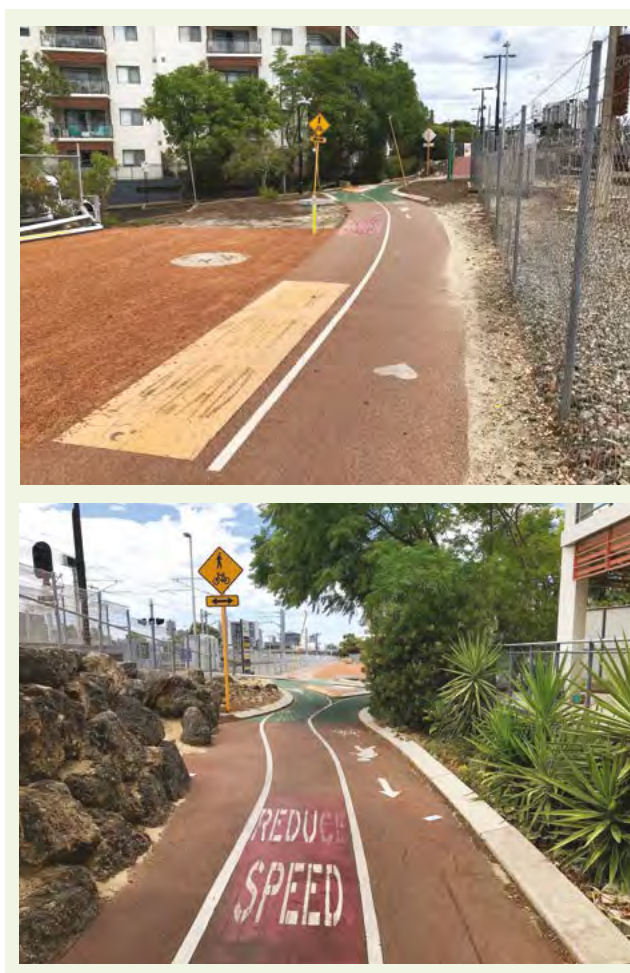
Figure 3.3 Entry point to shared zones, advisory measures are required to highlight the change of use/priority.
