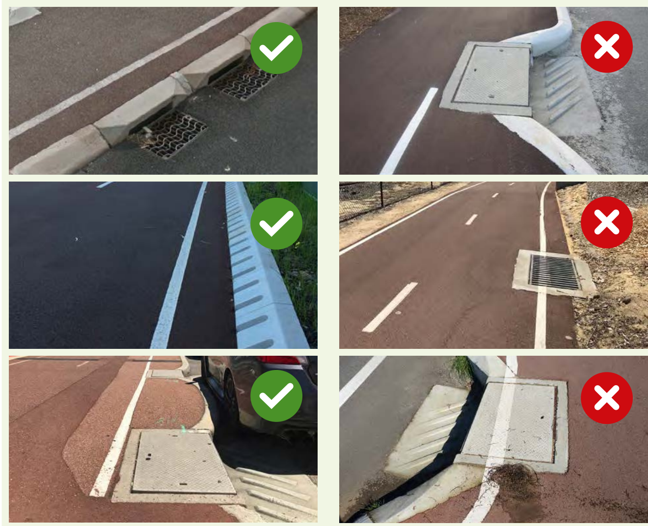
Figure 6.3 Examples of good and bad drainage applications.
