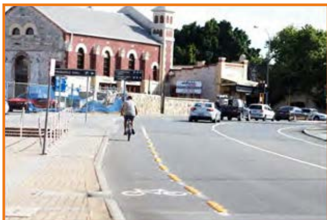
Bike lane separated by mountable plastic kerbing
