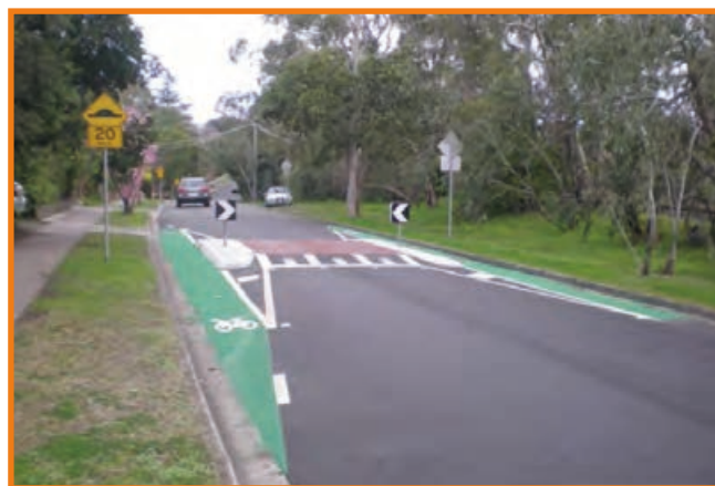
One-way slow point with bicycle-bypass facilities 3
