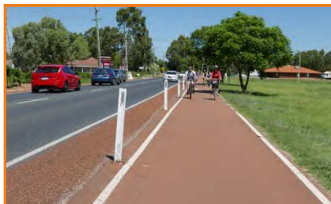
Bi-directional bike lane separated with bollards
