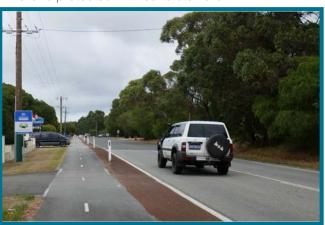
Bike lane separated with flexible plastic bollards
